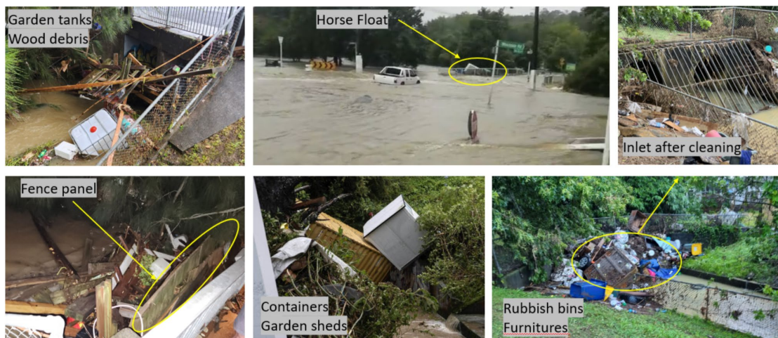
Figure 4. Records of culvert blockages during flooding events across the Auckland Region, prepared by HWFR
