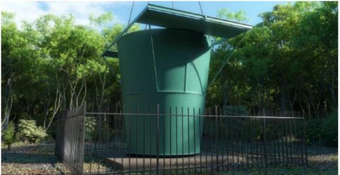
Figure 2-6 Typical air vent
