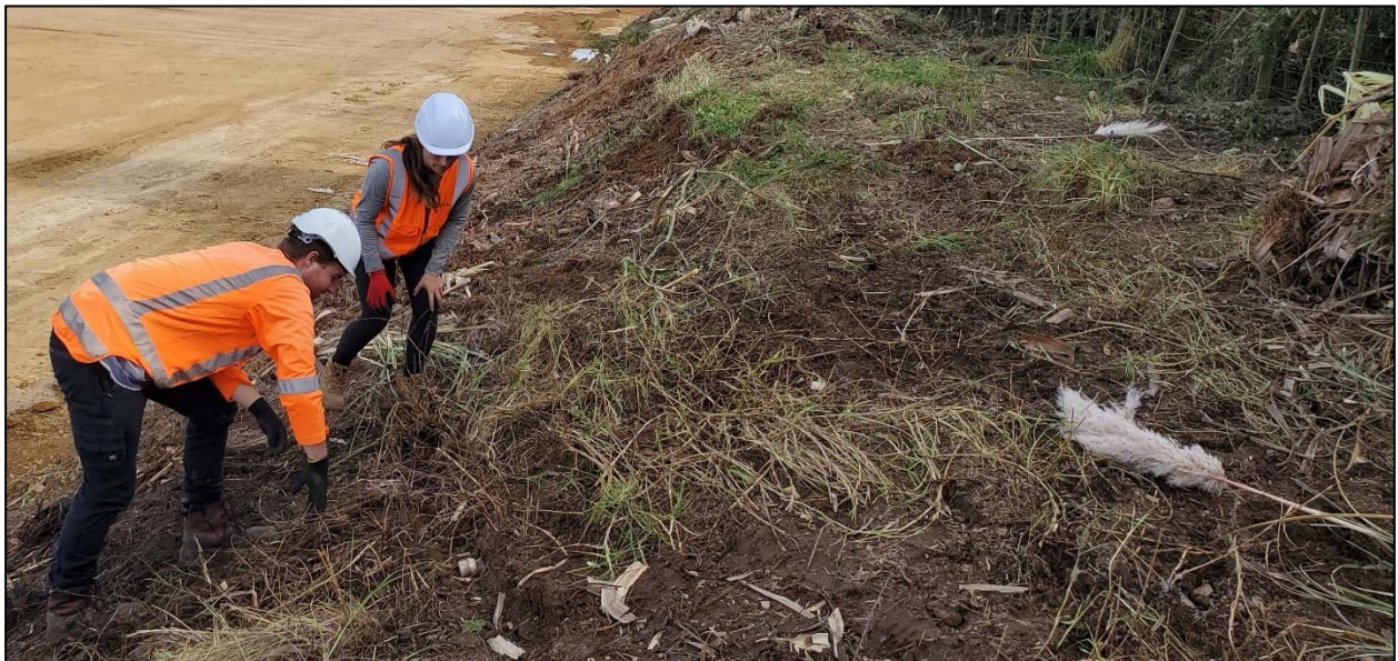
Photo 3: Post-works searching of clearance area
