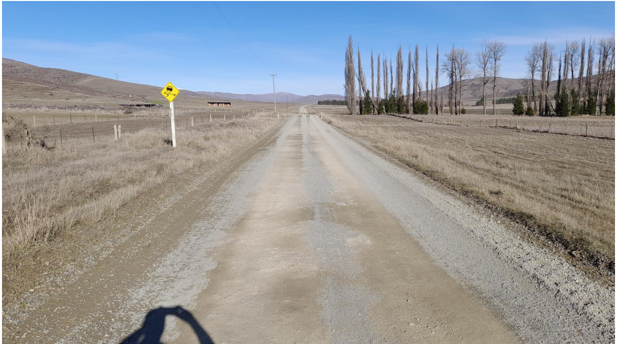
Figure 4-6: Typical Unsealed Section of Haldon Road
