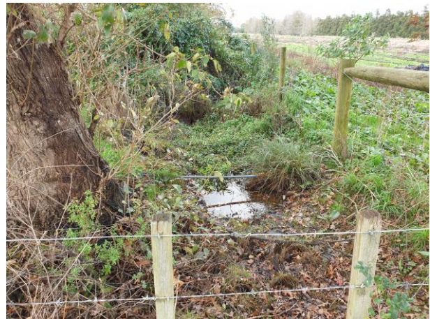
Photo 41. Drain k (northern reach)
