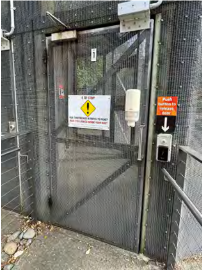
Predator free double gate allowing safe passage of pedestrians and dismounted cyclists in and out of predator-free enclosure
