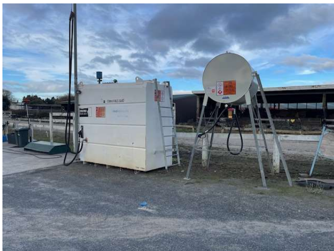
Photo 11: ASTs containing diesel and petrol
