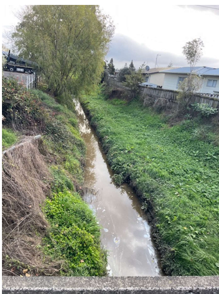
Photo 5: Lined open stormwater drain
