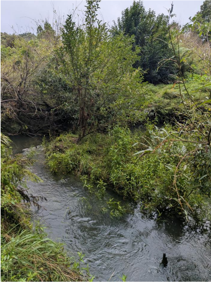
Figure 18. Example of flood chute activation following the storm event the week prior.
