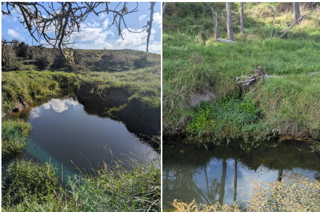
Figure 10. Geomorphic hotspot within Segment 1, outer meander erosion and inner bank slumping just downstream.
