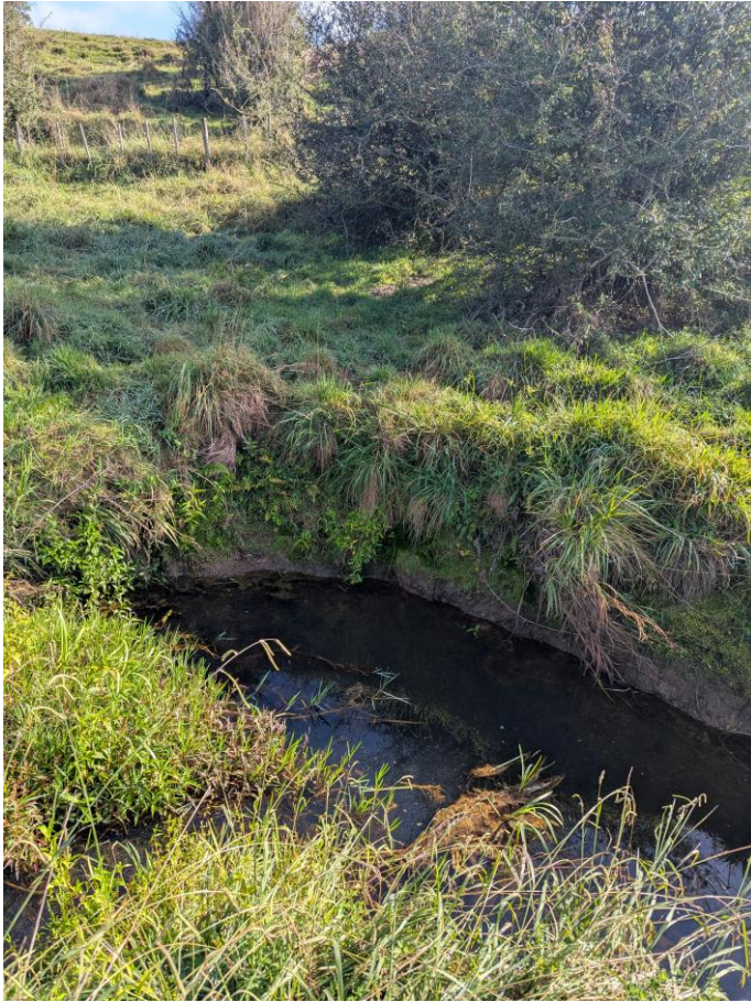
Figure 11. One of many locations indicating bank undercutting.
