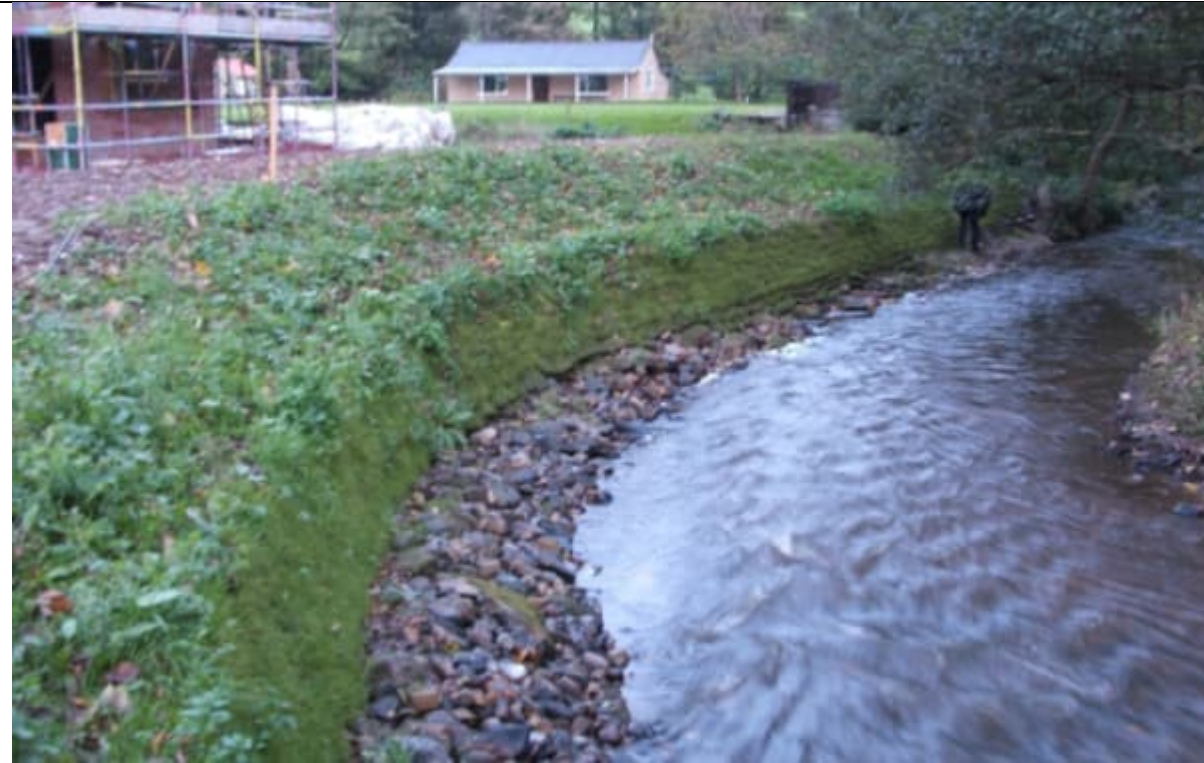
Combination riprap on lower banks and erosion mats on upper banks
