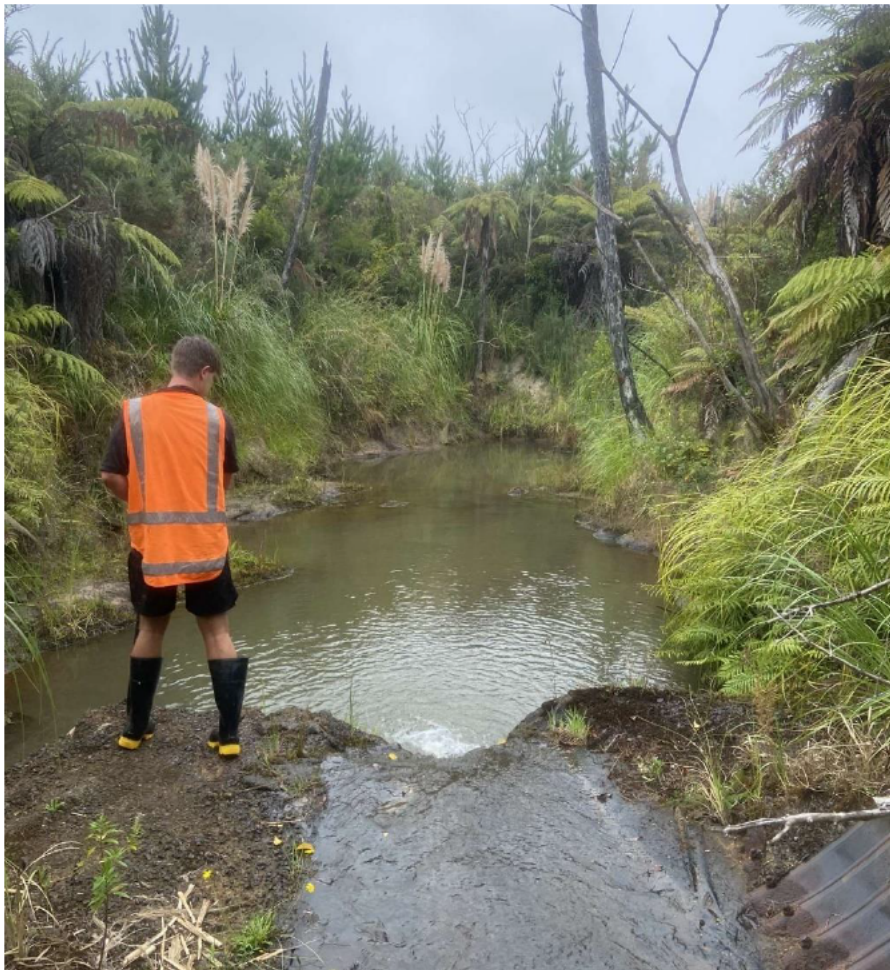
Figure 6 – example of a localised plunge pool caused by a culvert outfall.
