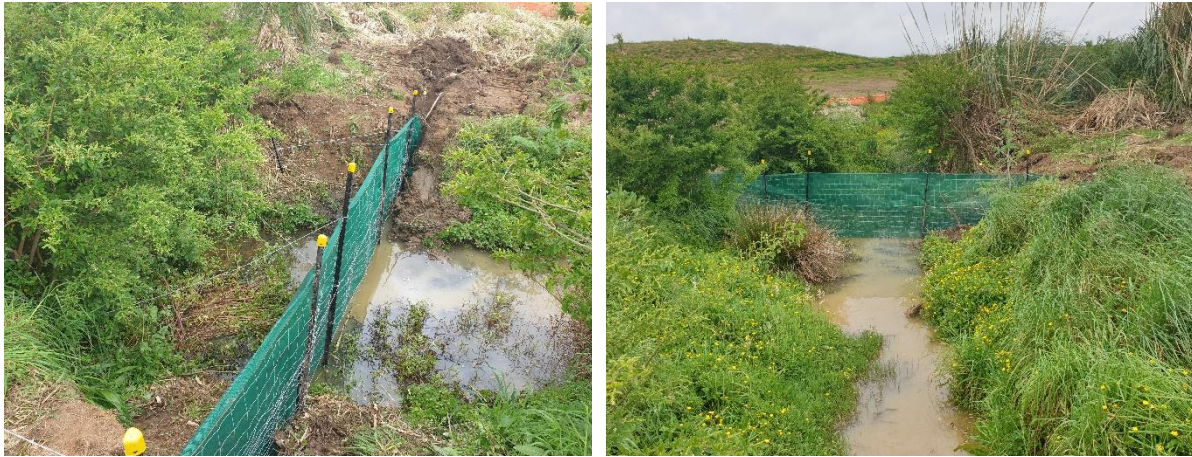
Photo 1 and 2. Photo examples of fish exclusion barriers
