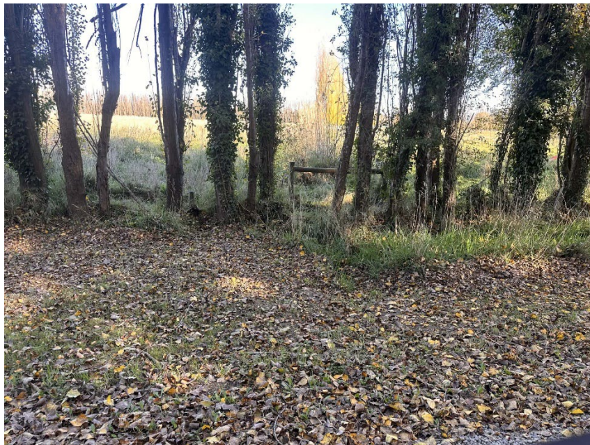
Location of existing Waihora Stream exiting 32 Jelfs Road on the right hand side of road and connecting with existing concrete culvert under Jelfs road.
