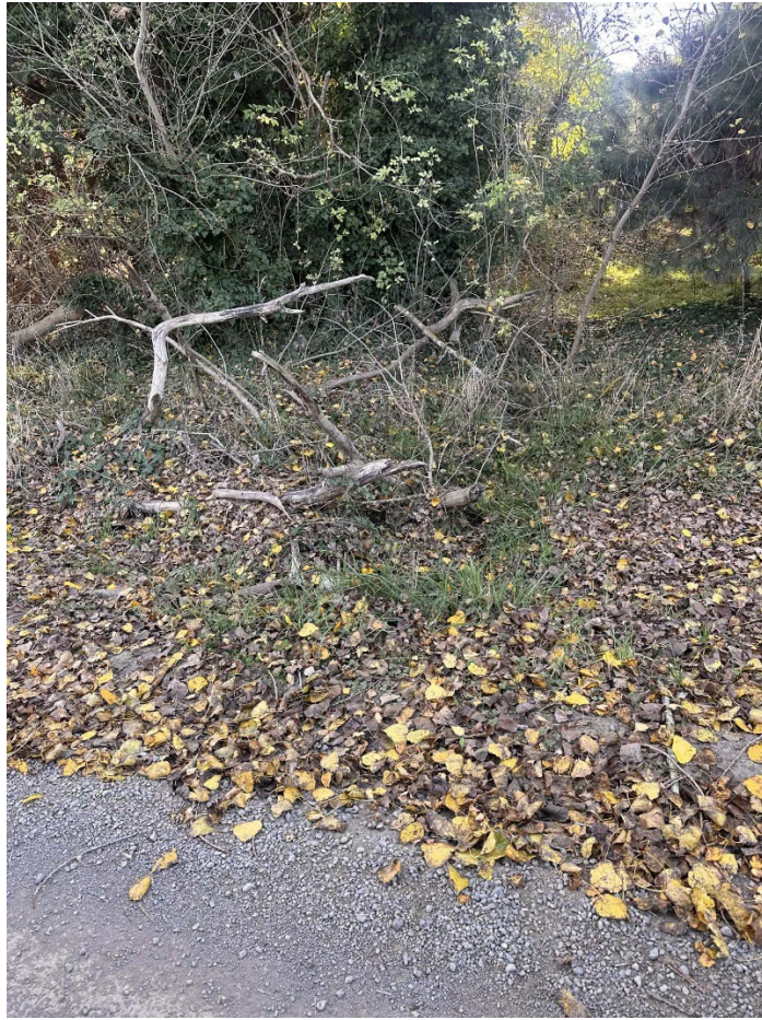
Location of existing Waihora Stream and culvert Jelfs Road. (Left Side)
