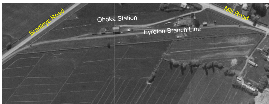
Figure 3: 1940-44 aerial image showing Eyreton Branch railway line Source: Canterbury Maps
