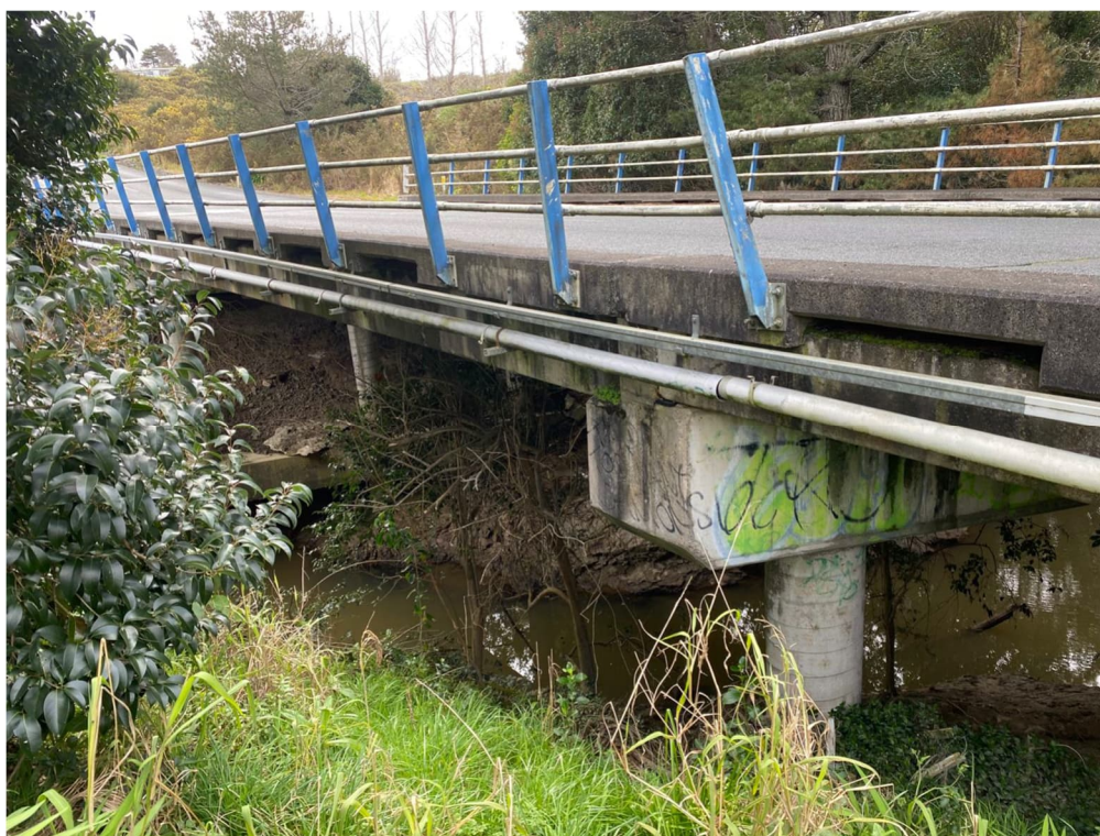
Figure 22: Upper Orewa Bridge side view
