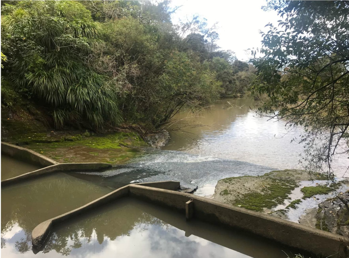
Figure 21: Kowhai Bridge downstream view
