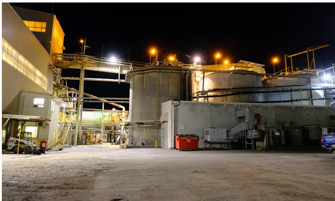
Figure 25: Processing Plant Area - Existing Lighting View 2
