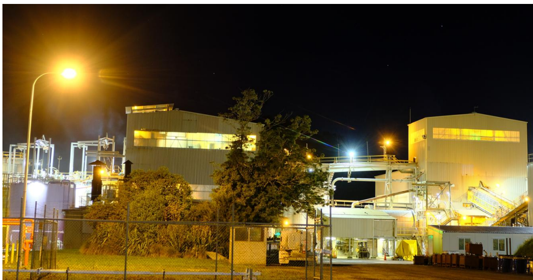
Figure 27: Processing Plant Area - Existing Lighting View 4
