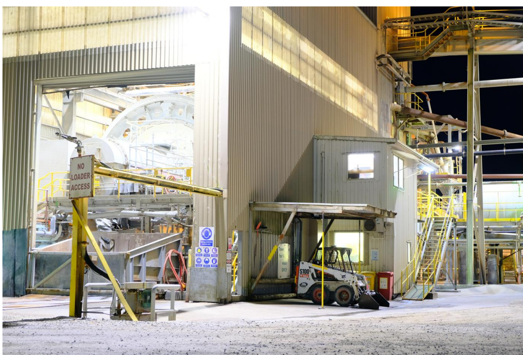
Figure 24: Processing Plant Area - Existing Lighting View 1
