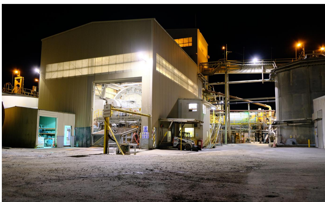
Figure 26: Processing Plant Area - Existing Lighting View 3
