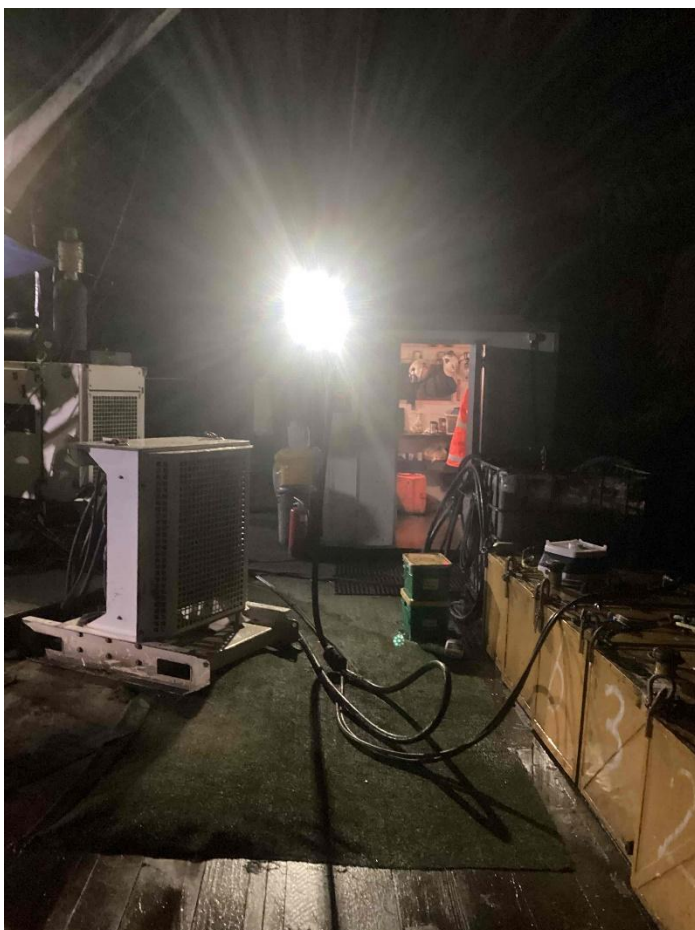
Figure 34: Drilling Site Lighting - Nighttime 2
