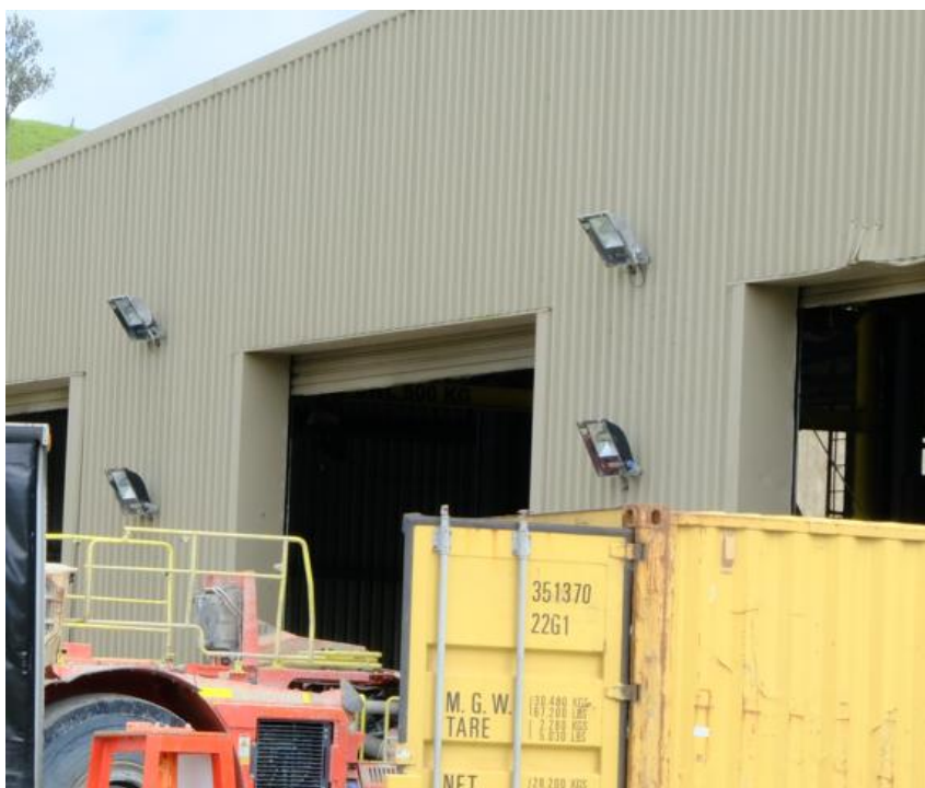
Figure 12: Existing Exterior Lighting Baxter Road Workshops
