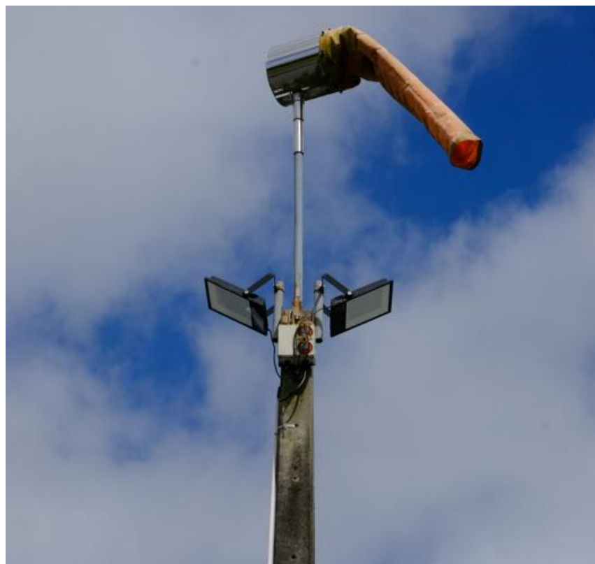
Figure 20: Typical Pole Mounted LED Area Light
