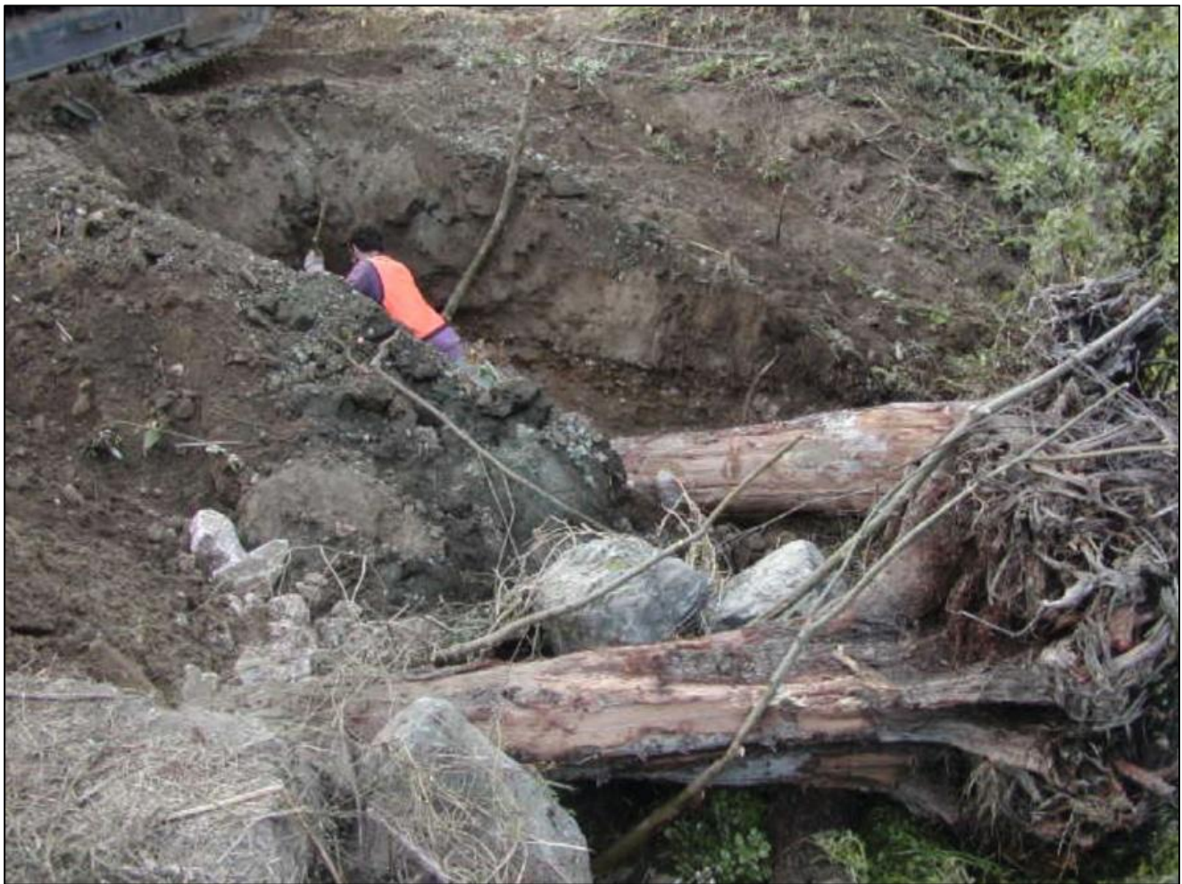
Figure 7: Root wads dug into stream bank and stabilised with boulders
