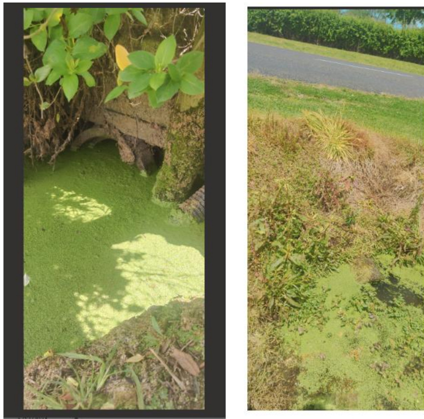
Figure 4: Existing Culvert with blockage Issue
