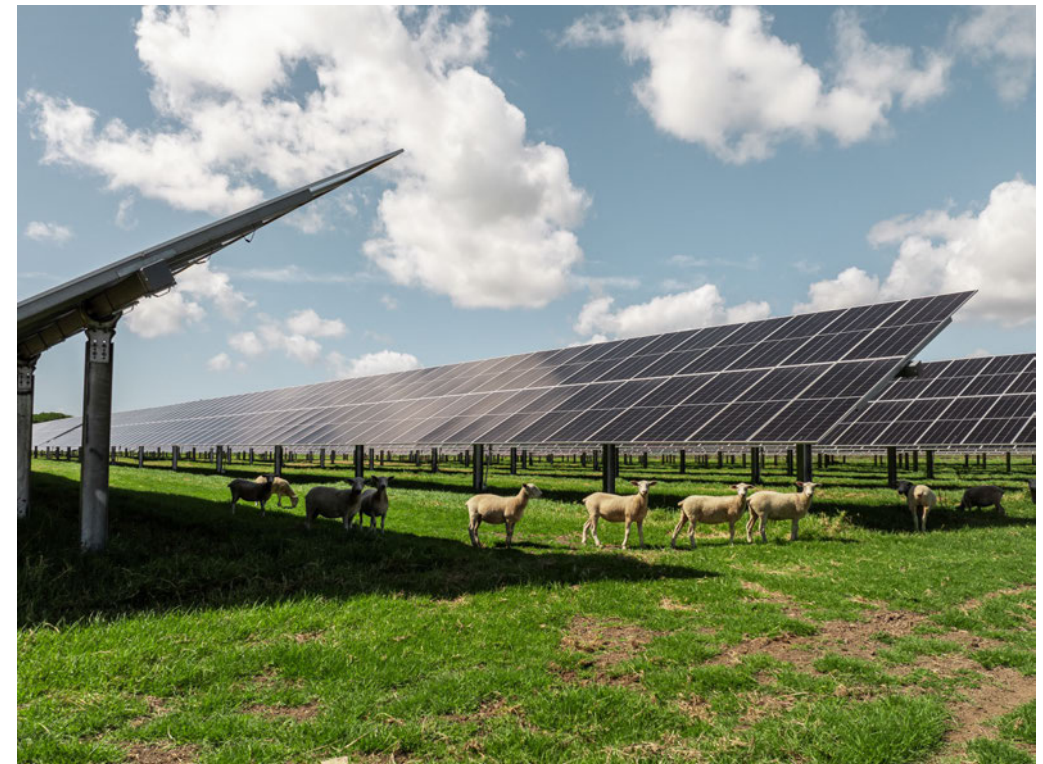
Trackers tilting to 55° to capture morning sun
