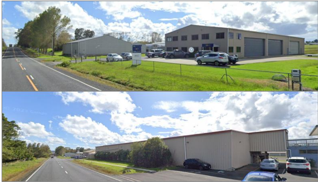
Figure 34: Buildings associated with the North Shore Aerodrome. Source: Google Images.
