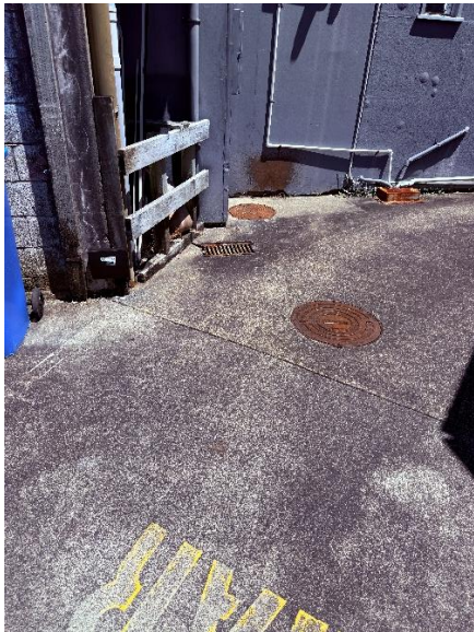
Figure 22: Modern services at the back of heritage buildings.
