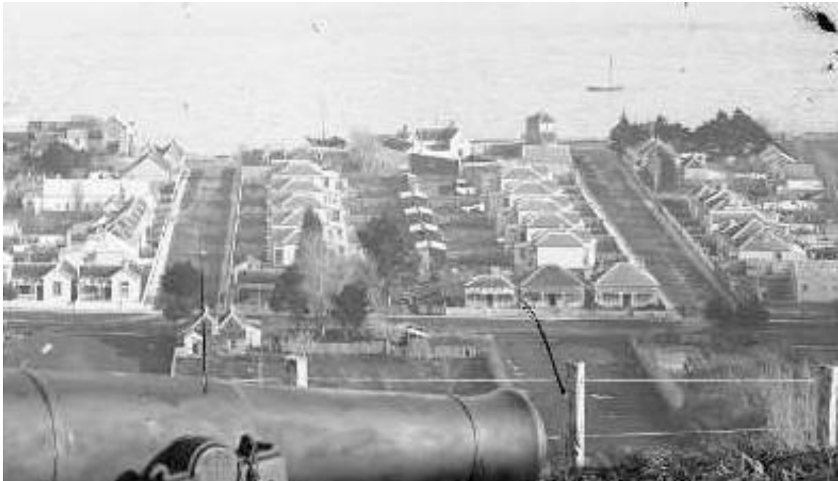
Figure 14: Detail of an 1880s photograph showing the ten identical buildings between Wynyard and Anne Streets (ATB 1_2-018635-G).
