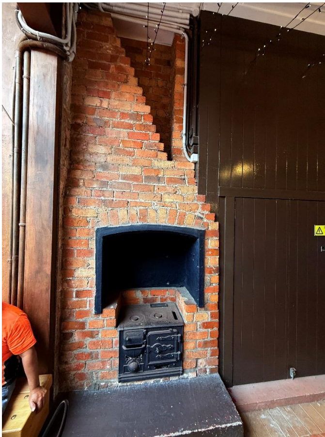
Figure 27: Kitchen fireplace displayed in the modern arcade opened up in the 1980s, dating back from the infill of the arcade in the early 20 th century.
