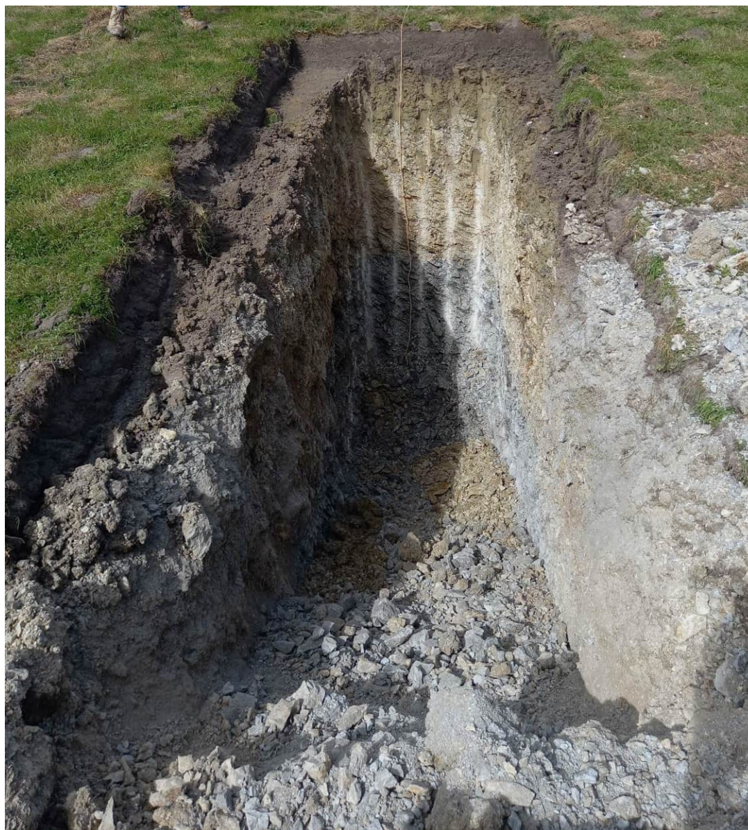
TP01-23 – TEST PIT EXCAVATION
