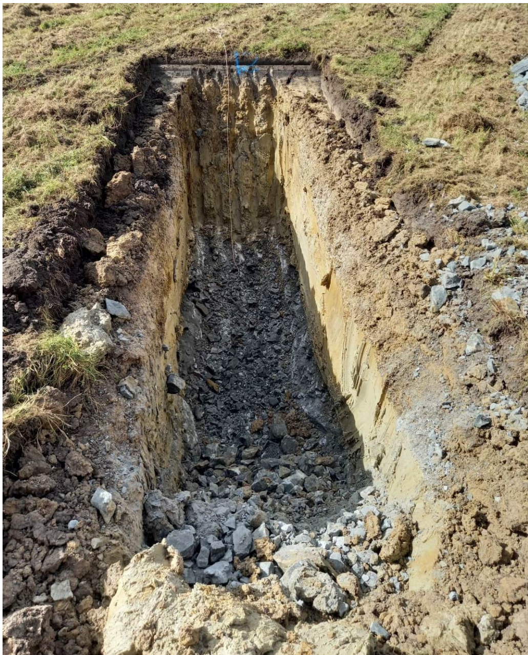
TP12-23 – TEST PIT EXCAVATION
