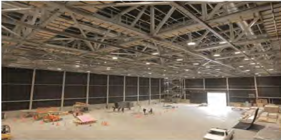
04 Kumeu Studio in construction
