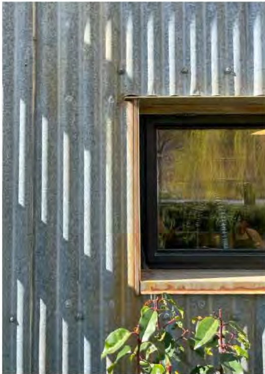
Corrugate cladding on the Woolshed
