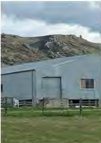
Slats to the undercroft
