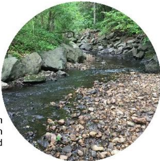
Right: Riffle created with gravel, rock armouring in background
