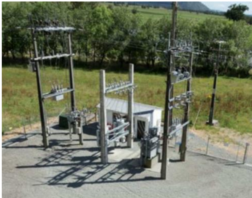
Figure 5 – Indicative Example of Switching Station
