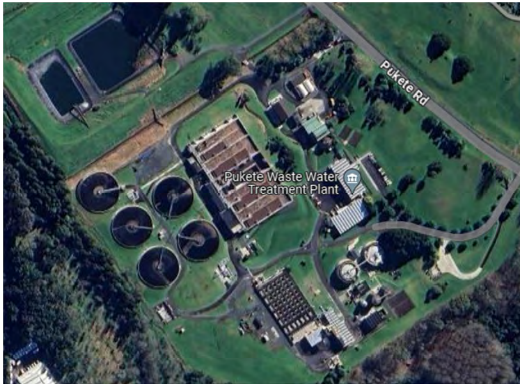
Figure 9 - Pukete Wastewater Treatment Plant (Google Map)
