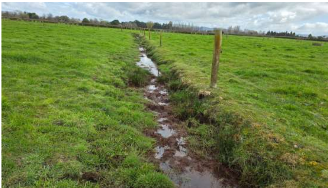
Figure 18. One of the many drainage ditches within the lower flat area of the Site.
