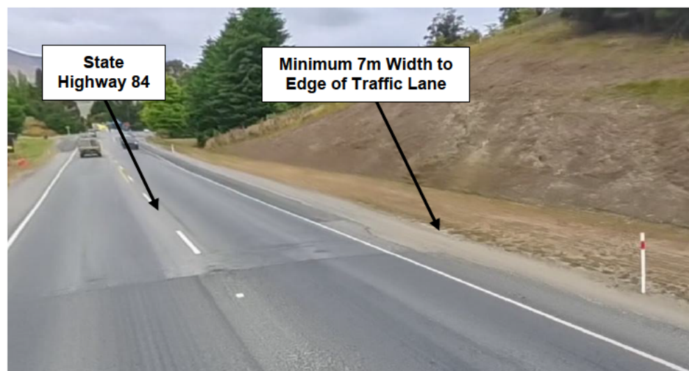
Figure 2: Adequate Width between Toe of Bank and Movement Lanes (Source: Google Streetview)
