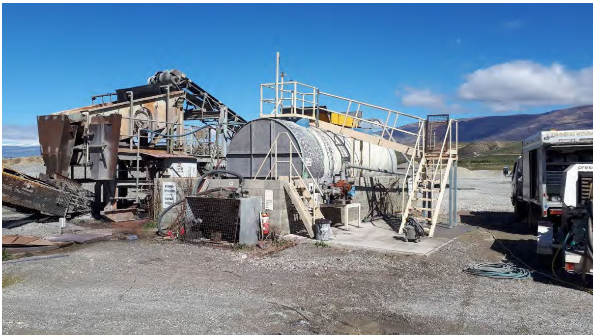
Figure 6: Bitumen spray plant within quarry.
