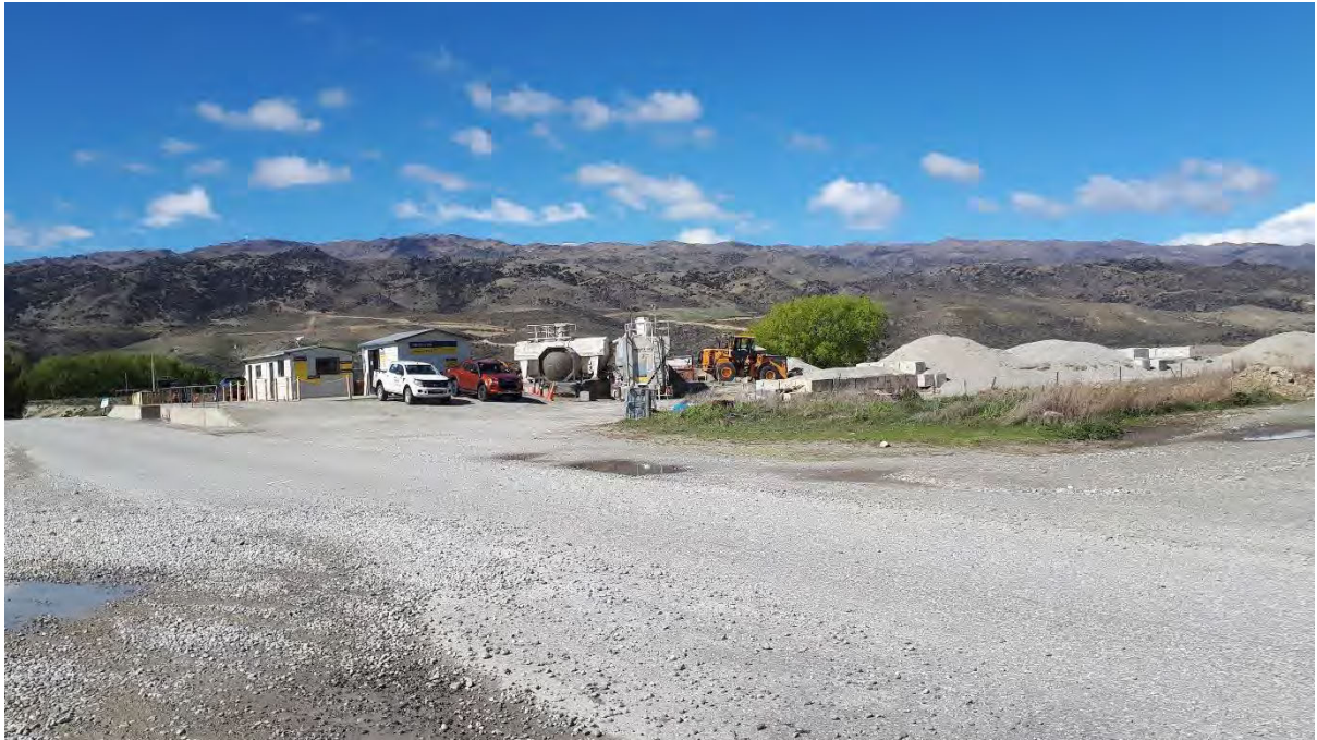
Figure 13: Allied concrete batching plant.
