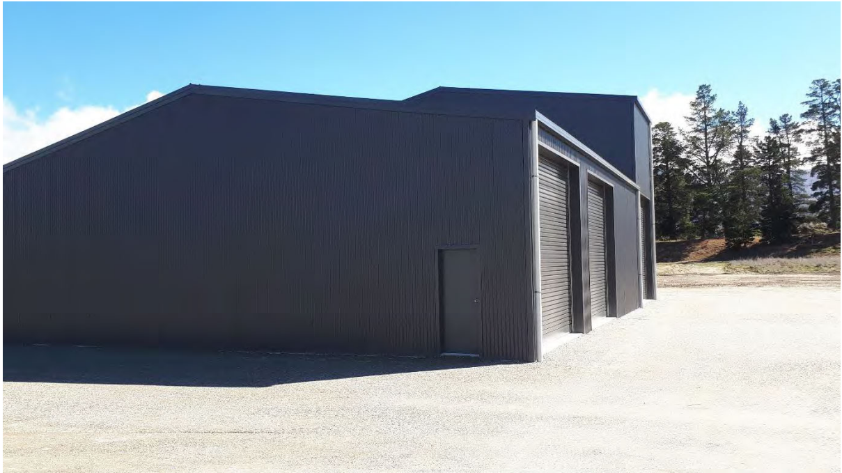
Figure 19: New glass processing building.
