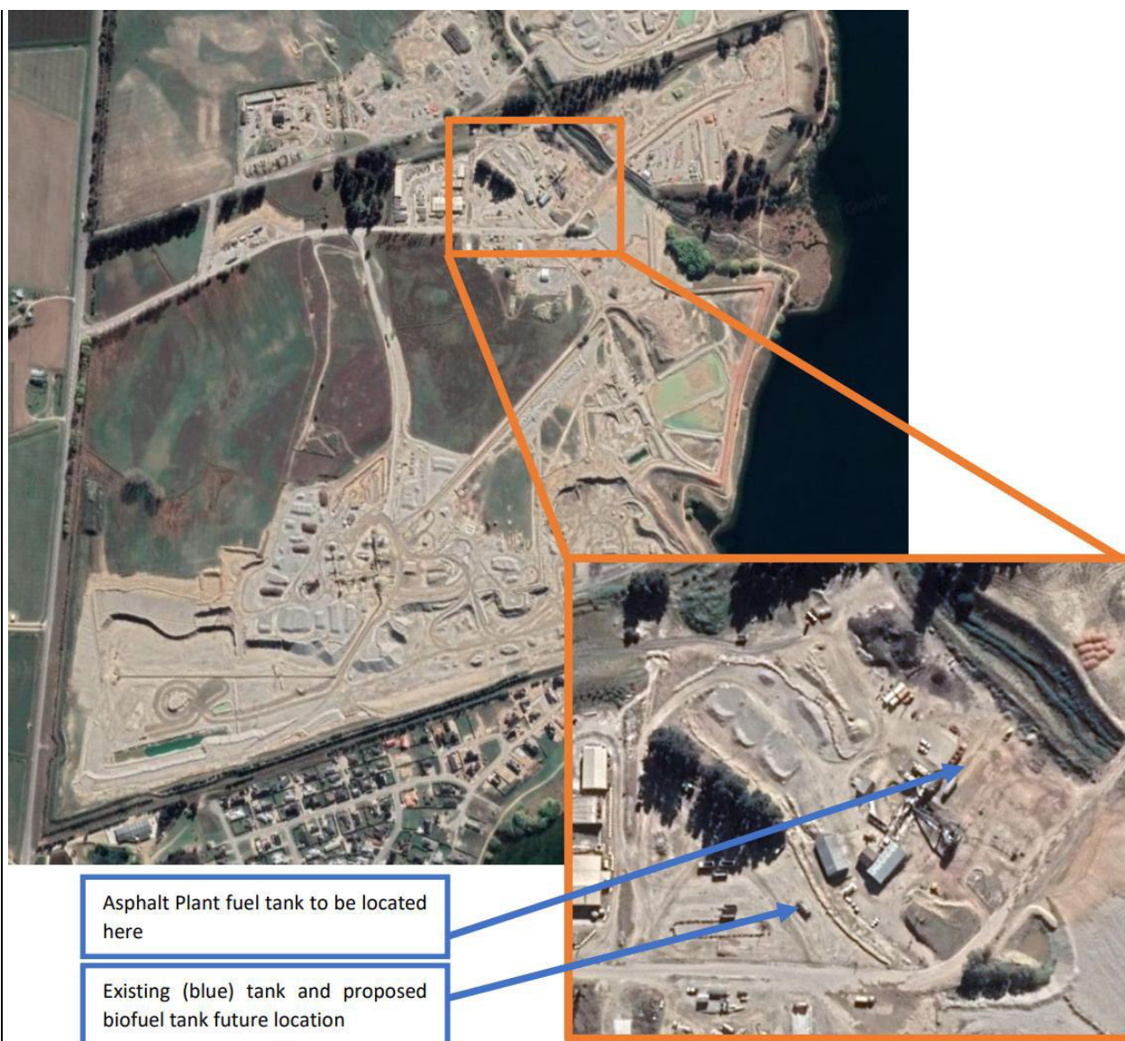
Figure One: Extract from application for RC 210129 showing location of pre-existing and proposed fuel tanks.
