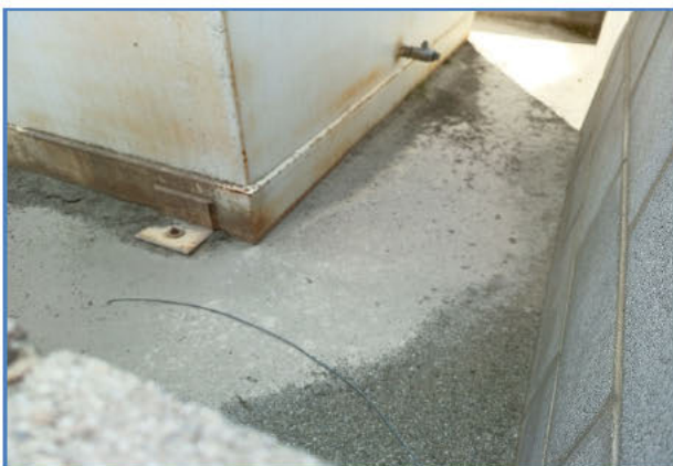
Photo 2: No evidence of petroleum hydrocarbons in the bunded area.
