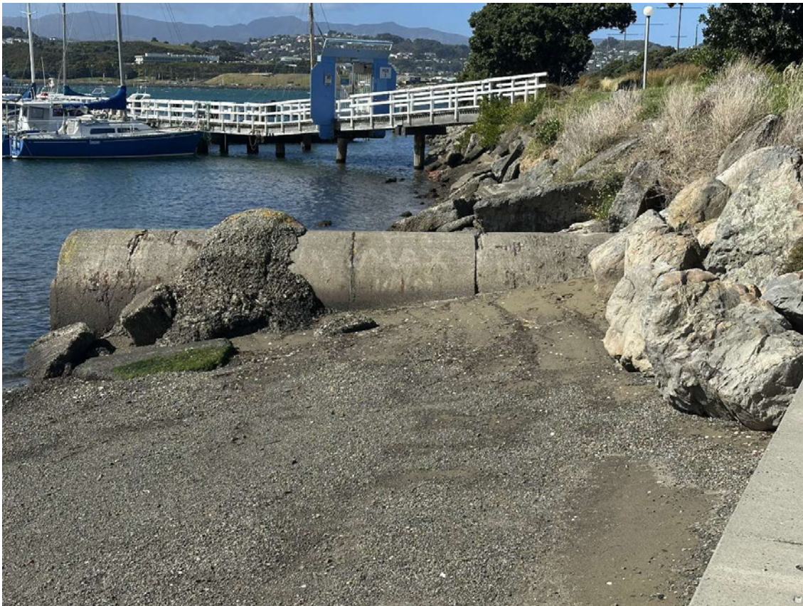
Figure 4 - Evans Bay stormwater outfall looking East, including the fine sediment/gravel beach to the west of the stormwater outfall
