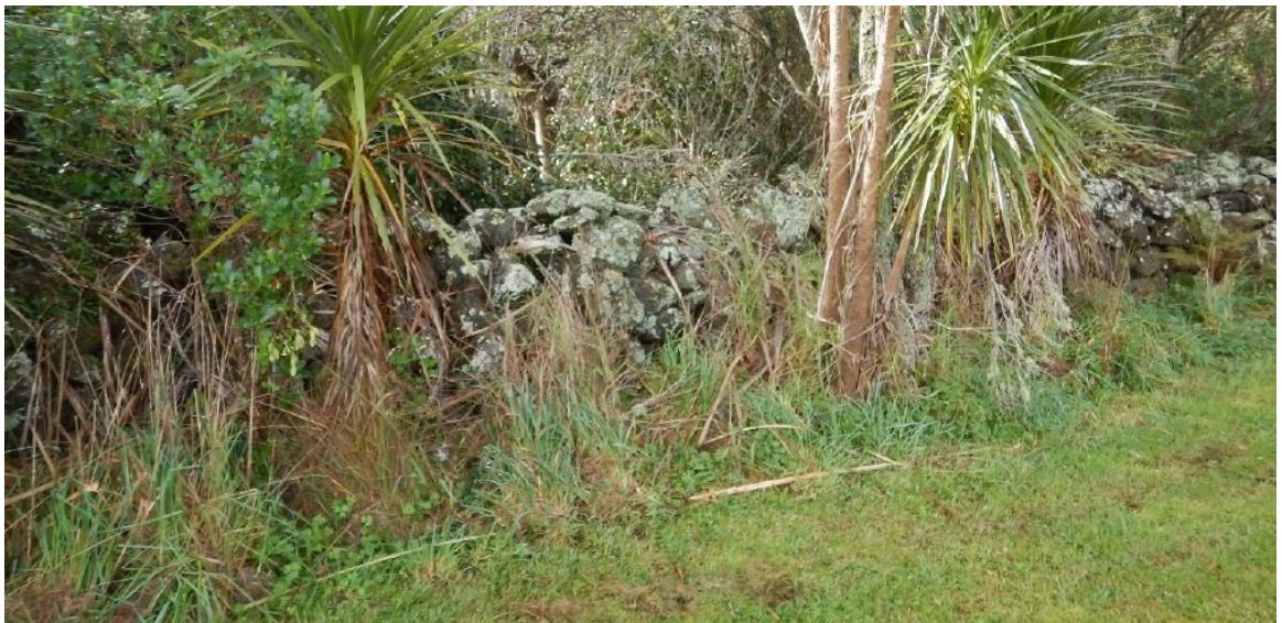
Figure 22. Photograph showing the northern part of the drystone wall (R10/1452) in 2015, looking east
