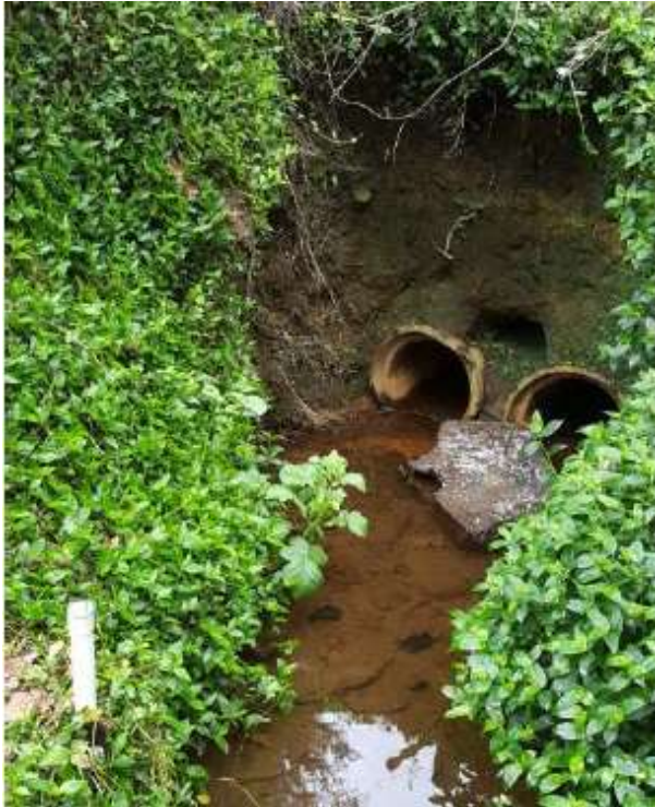
Figure 2 TB4 monitoring location upstream of culvert
