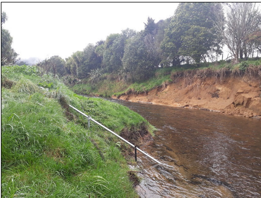
Figure A.2 Surface water level monitoring site installed in Ohinemuri River
