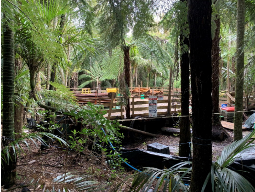
Figure 17. Existing Drill Site 1 at the Wharekirauponga Mining Area
