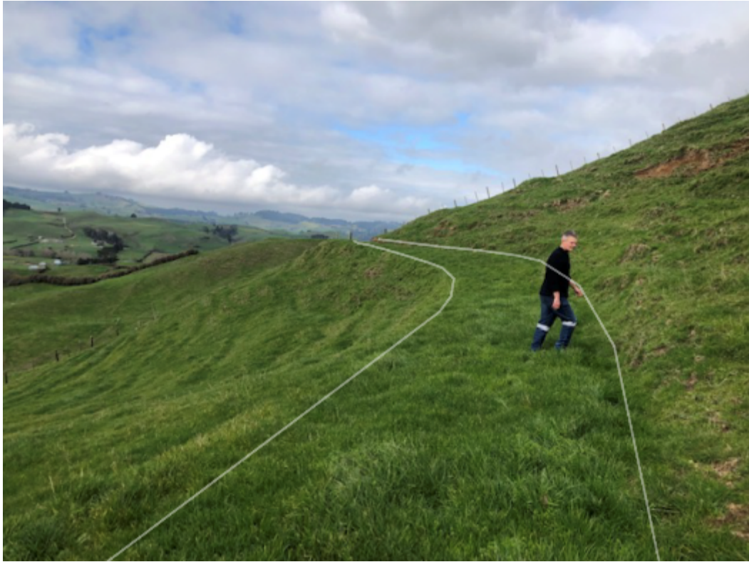
Figure 39. Looking along a section of the High-Level Walmsley Timber Tramway alignment above and west of the portal. This section has been widened as a farm track (alignment highlighted in white)
