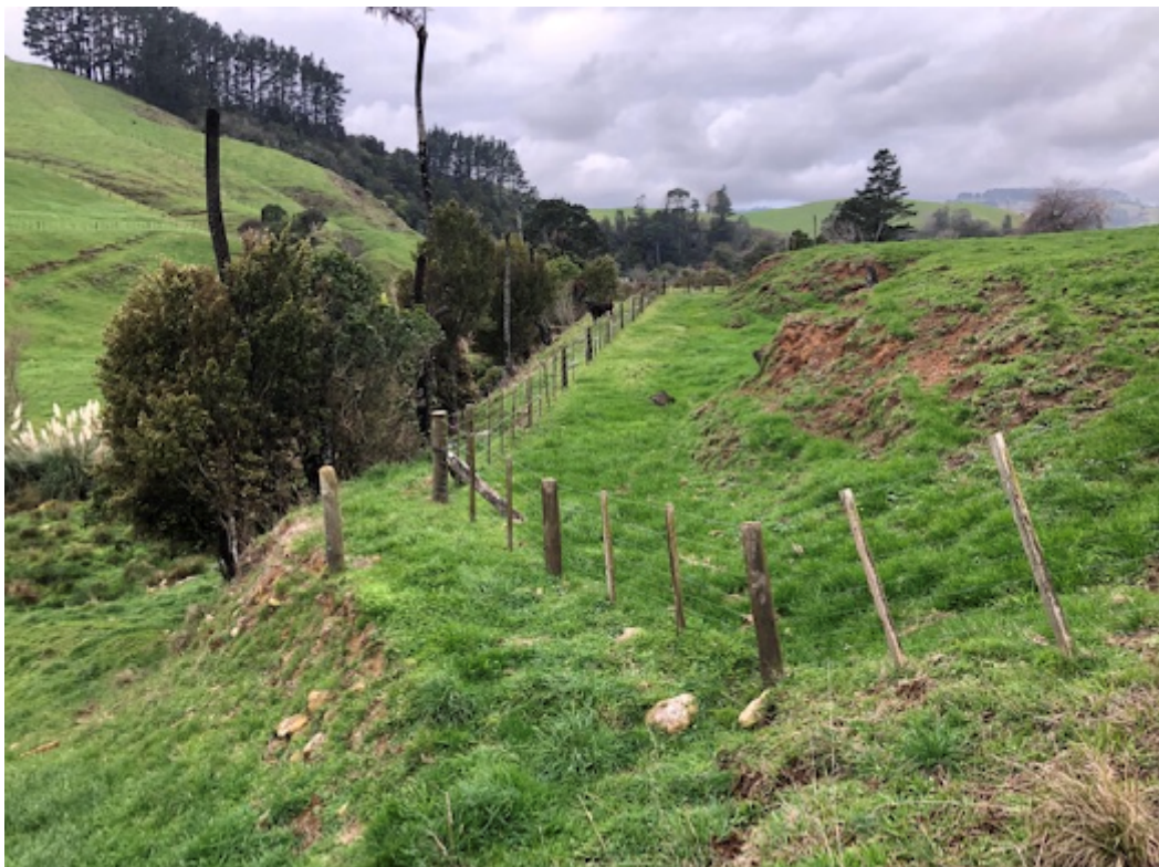
Figure 34. Water race alignment visible as a levelled or benched track alongside the Mataura Stream
