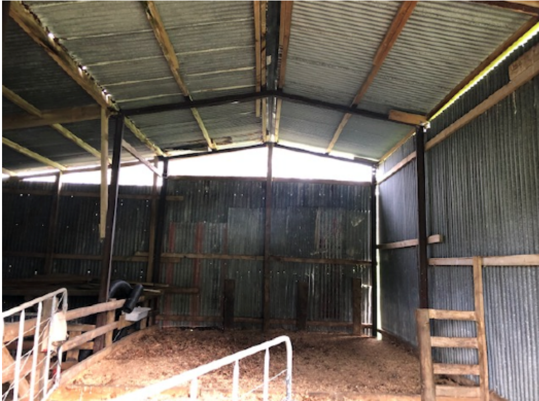
Figure 37. Interior of the barn with structural beams made of tramway rails from the Willows Timber Tramway
