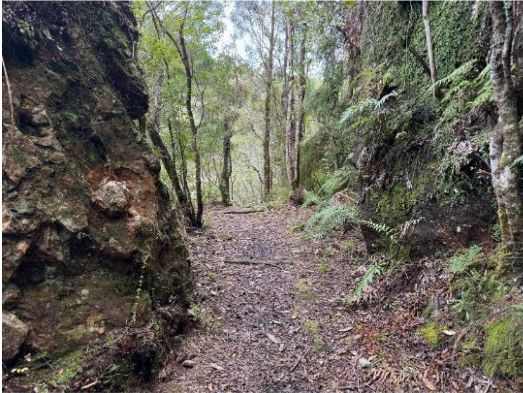
Figure 12. Deep cutting on the Lower Tramway Track (T12/681)
