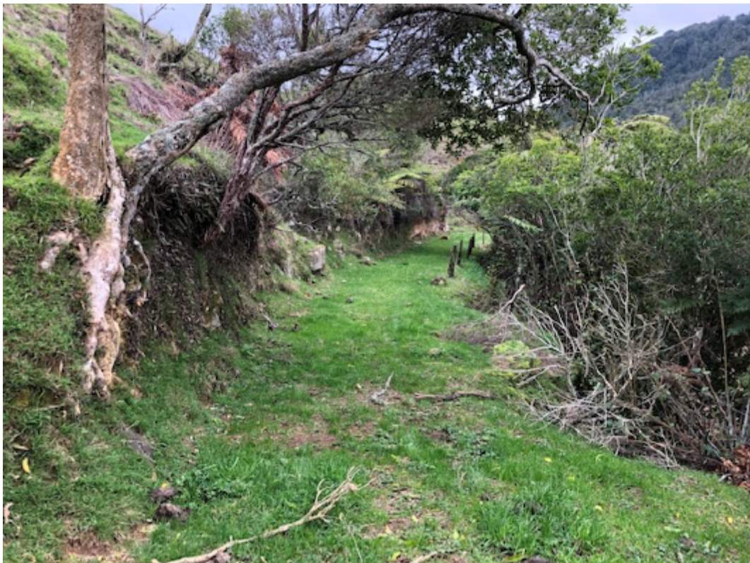
Figure 30. Mataura Water Race alignment near its intake on the Mataura Stream visible as a levelled or benched track
