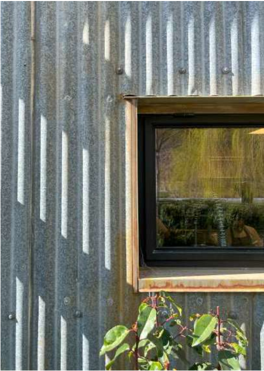
Corrugate cladding on the Woolshed
