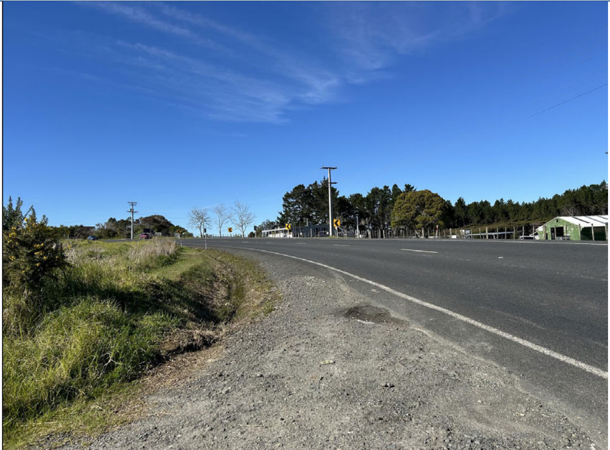
Figure 1: Sight line for Access 1 towards the east, showing grass within the legal road obstructing visibility
