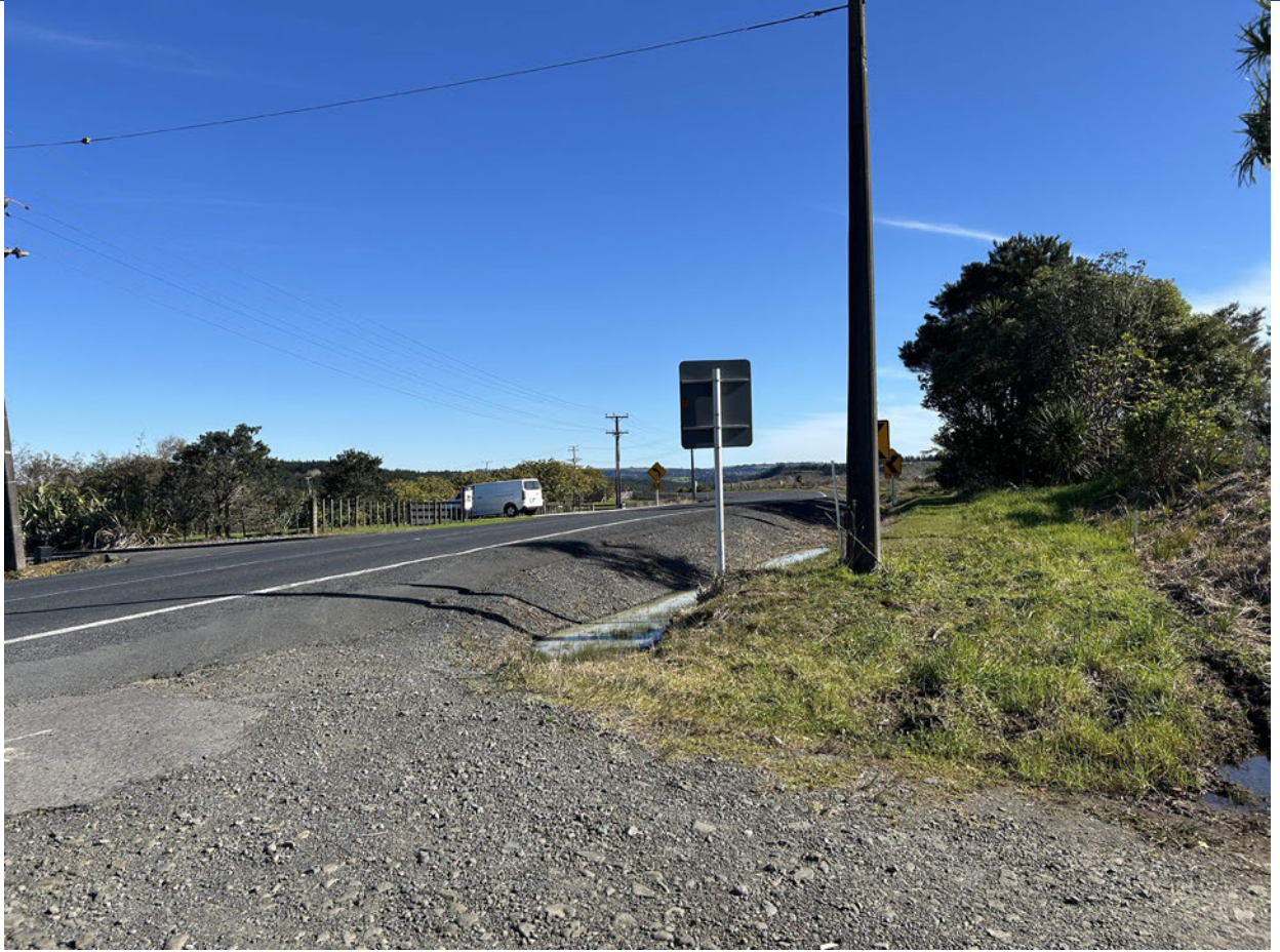
Figure 3: Sight line for Access 2 towards the west, showing sight line obstruction by existing fencing
