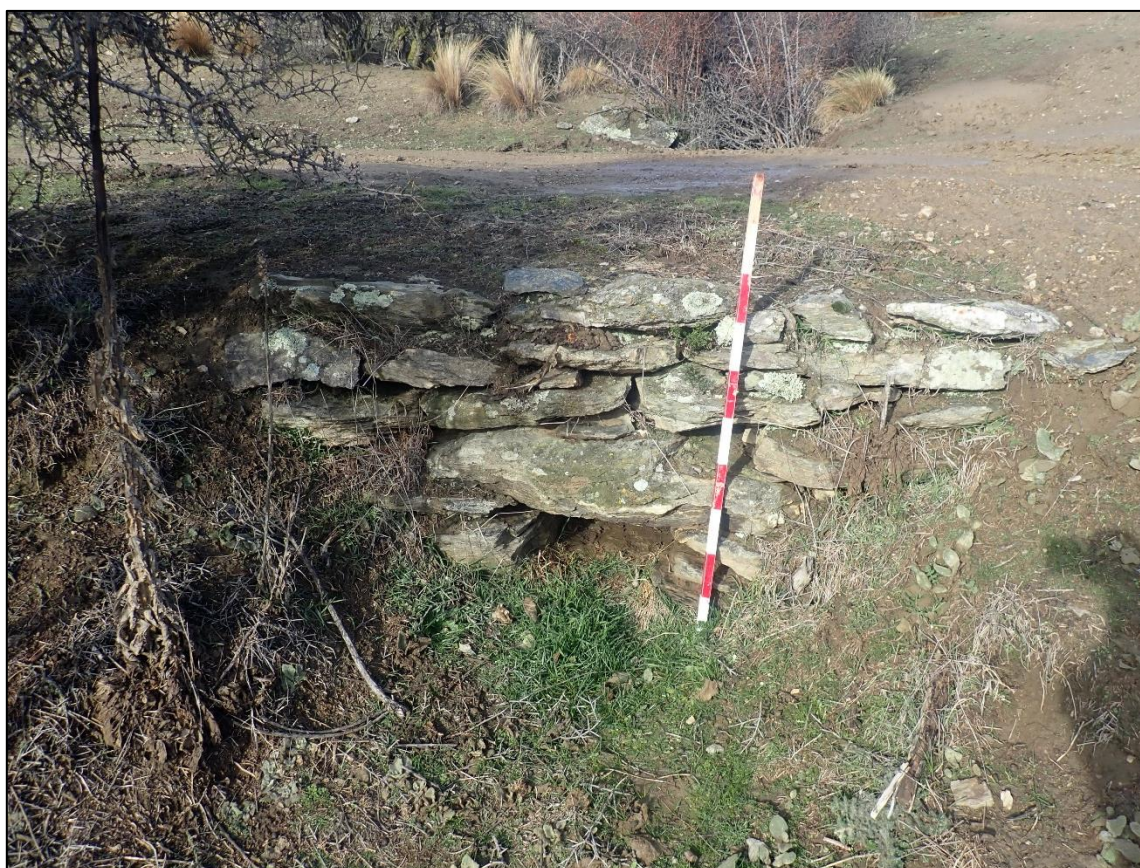
Figure 8. Photograph of culvert (POI 798) looking north.
