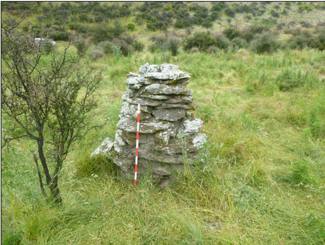
Figure 4 Photograph looking southwest at chimney recorded as G41/678. Photograph taken by Phoebe Scrivener on 19/12/18.
