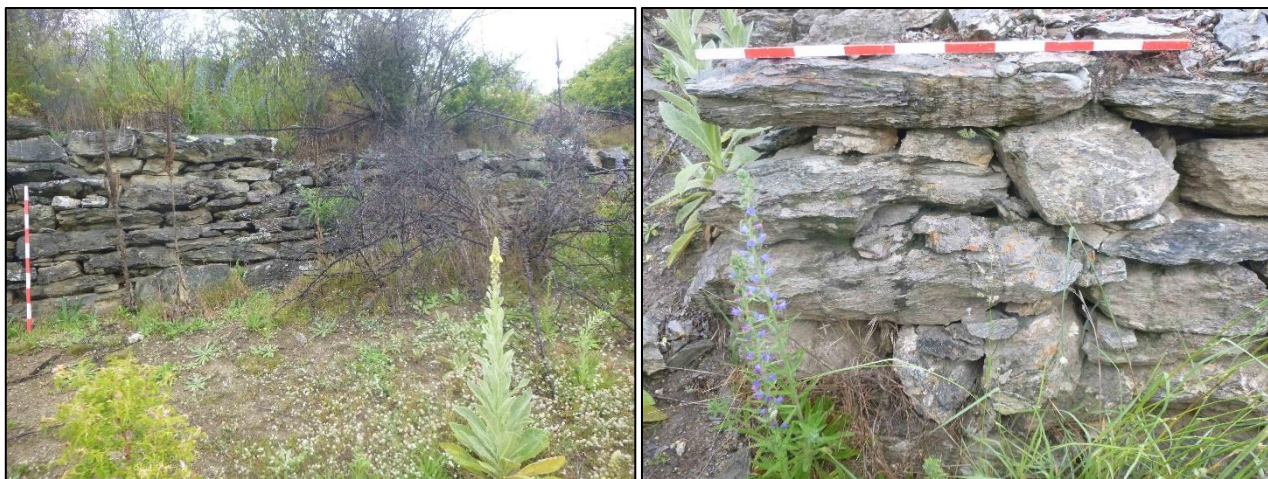
Figure 7. Photograph looking south at stacked schist revetment (POI 241-243).
