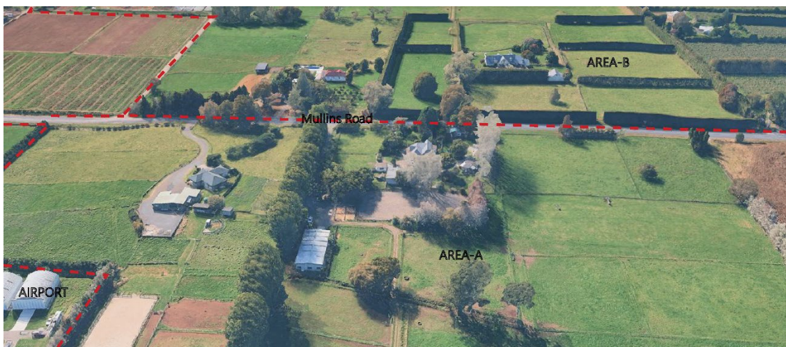
Figure E - View from above Area A looking east with Mullins Road horizontal through the image, Area B at the top, and Area A on the bottom (image Google Earth).
