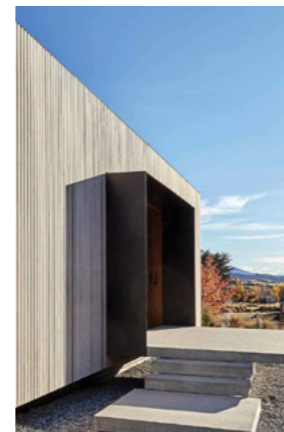
Raised built platform to account for level changes
