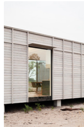
Timber weatherboards with raised batten detail
