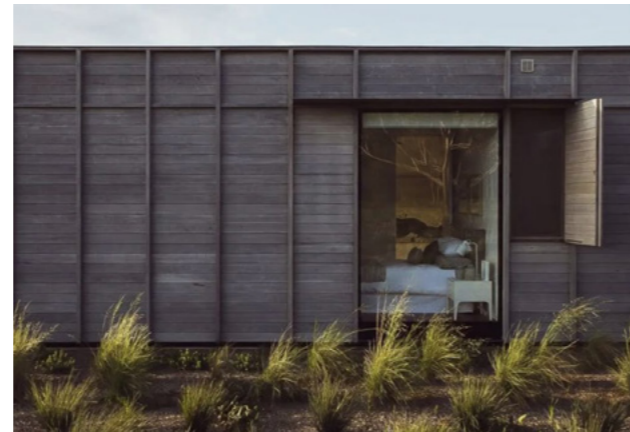
Timber weatherboards with raised batten detail
