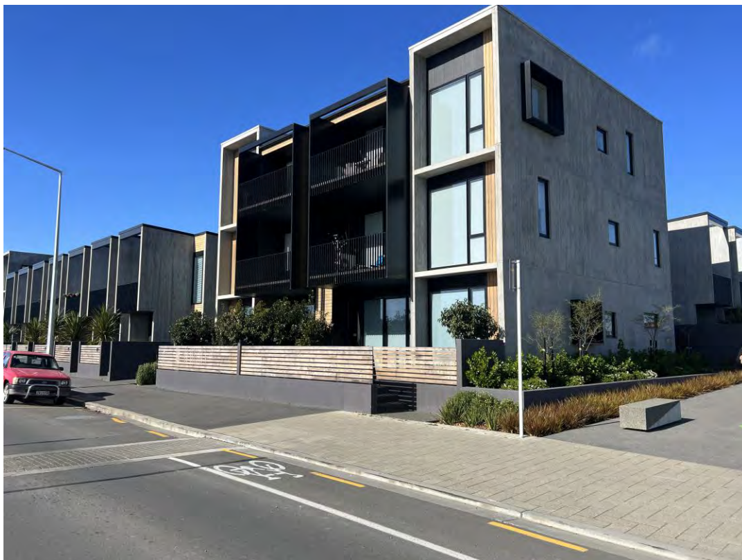
Figure 2 – The photo above is of a Sheppard and Rout design for a 3-level apartment building in the East Frame Christchurch. The units are orientated to the north, overlooking Gloucester St with the western, corner façade punctuated by windows at irregular spacings.
