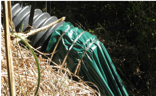
FIGURE 7: TYPICAL CULVERT / FLUME CONNECTION DETAIL
