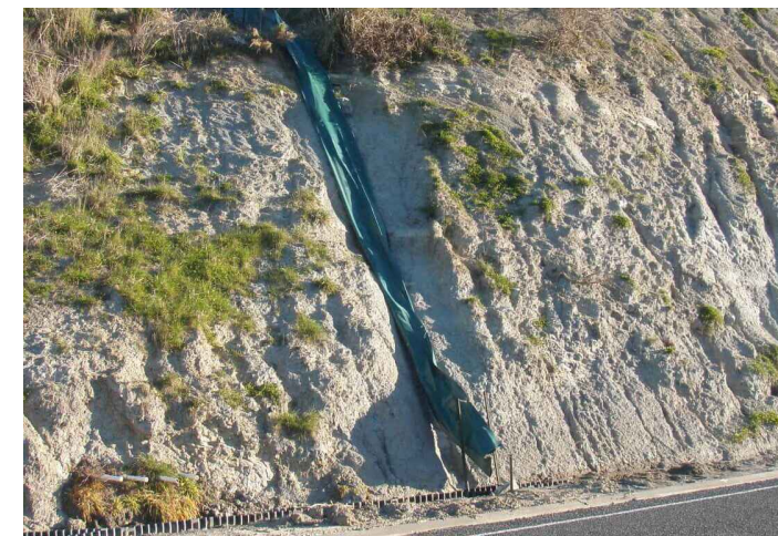
FIGURE 13: TYPICAL FLUME INSTALLATION
