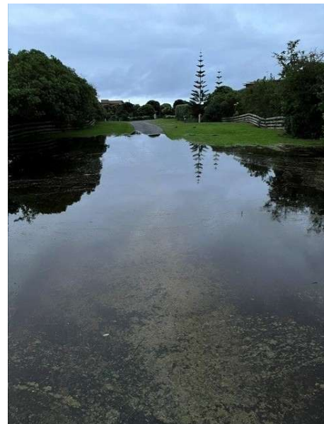
Floodwater blocking the only vehicular access to six Paetawa Road properties
