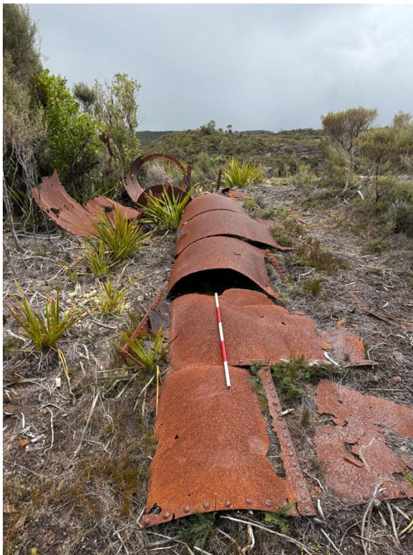
Figure 22. Broken metal remains of the vertical chimney at the top of the brick reclining airway/chimney of the Kiwi Mine Fan House and Compressor
