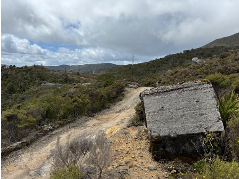
Figure 15. Features 207/208, Return Airway concrete pillar/foundation located above and south of the road at its intersection with the pylon road
