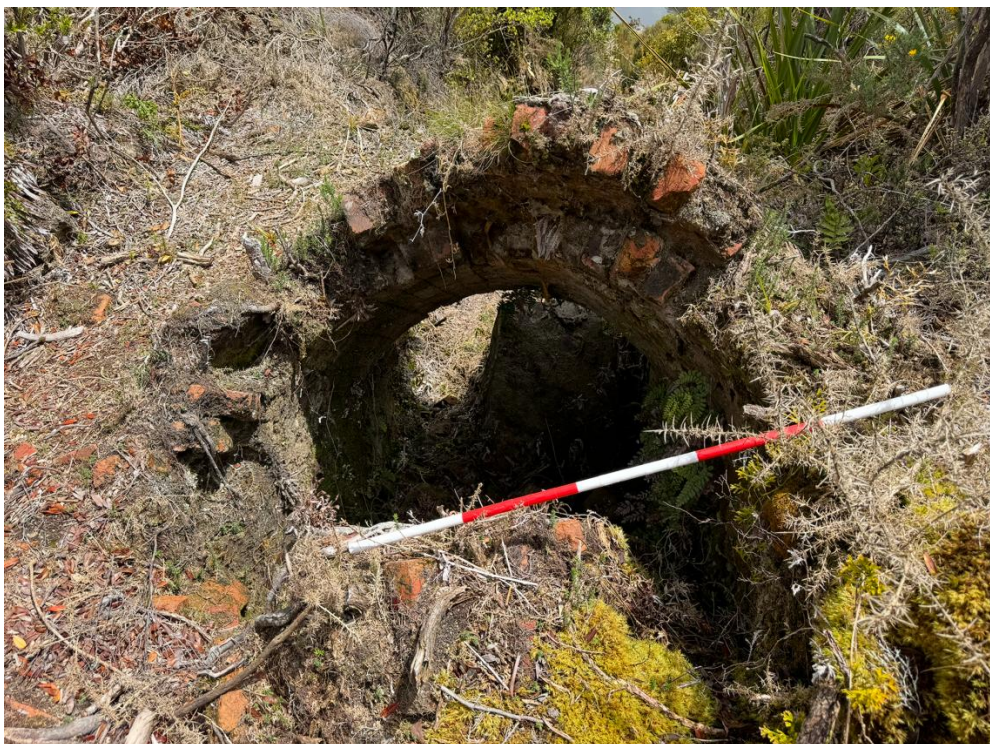
Figure 20. A partially intact section of the Kiwi Mine Fan House and Compressor brick reclining airway/chimney
