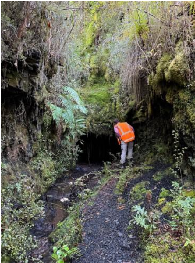
Figure 24. Northerly mine entrance at Beggs Outcrop
