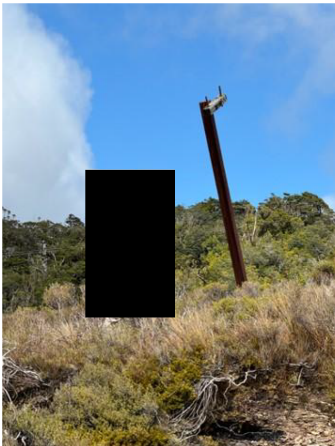
Figure 18. A power pole located immediately above Cedar Creek Road and the proposed UWHR construction corridor
