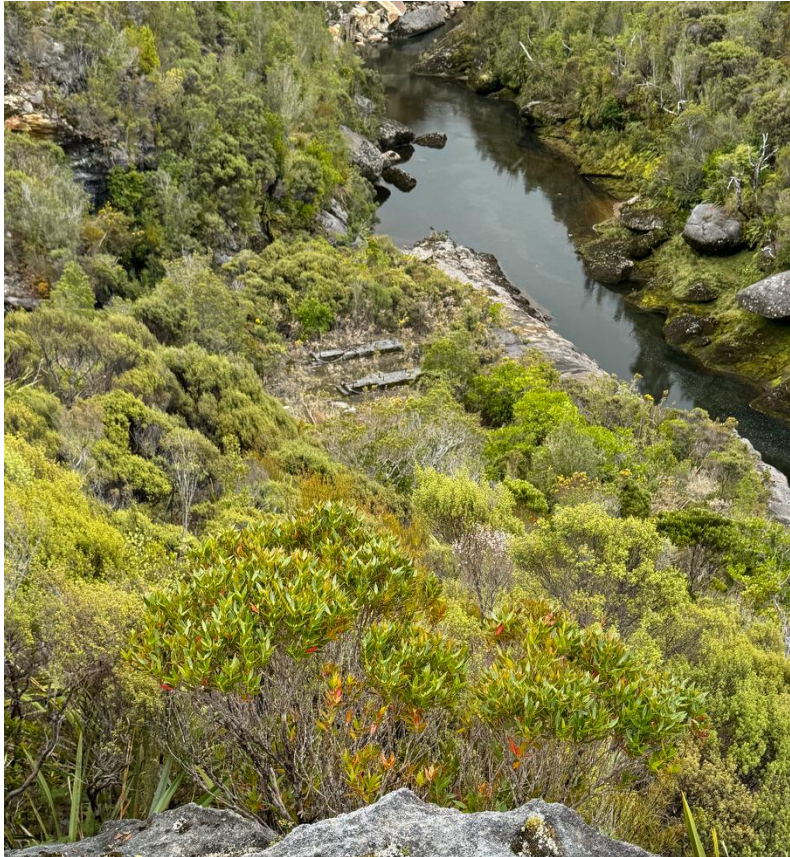
Figure 19. Looking down from the top of the reclining chimney to the power house and machine concrete foundations of the Kiwi Fan House and Compressor
