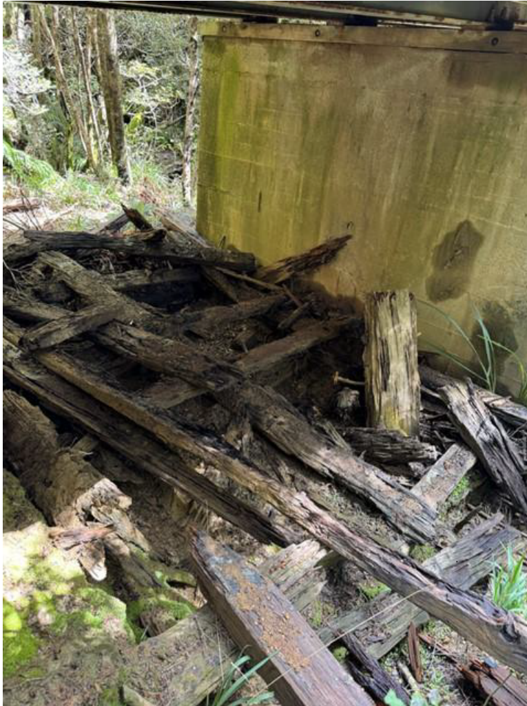
Figure 29. Features 225/226 beneath the modern road bridge are the discarded bearers and timbers of an earlier bridge
