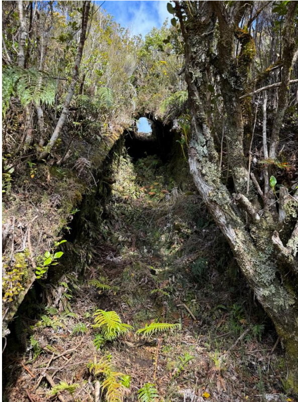
Figure 21. Looking up along a collapsed section to the top intact of the Kiwi Mine Fan House and Compressor brick reclining airway/chimney
