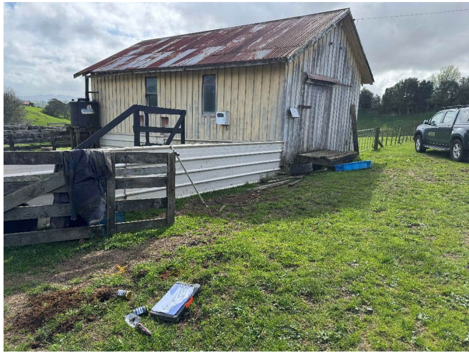
Photo 19: Storage shed within Stockyard 1 (1 October 2025).
