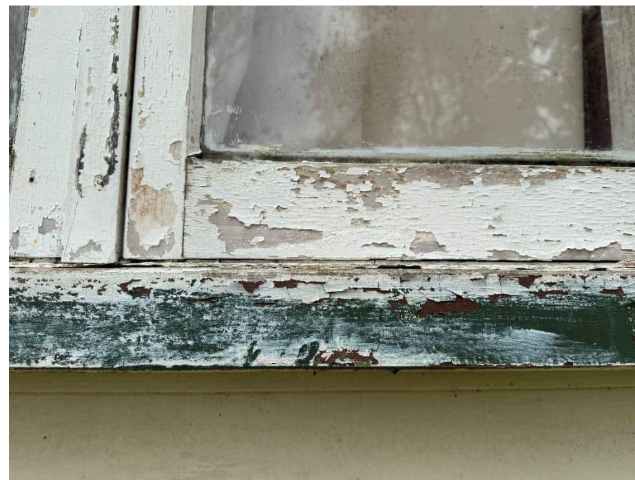
Photo 11: Degradation of potential lead-based paint (1 October 2025).
