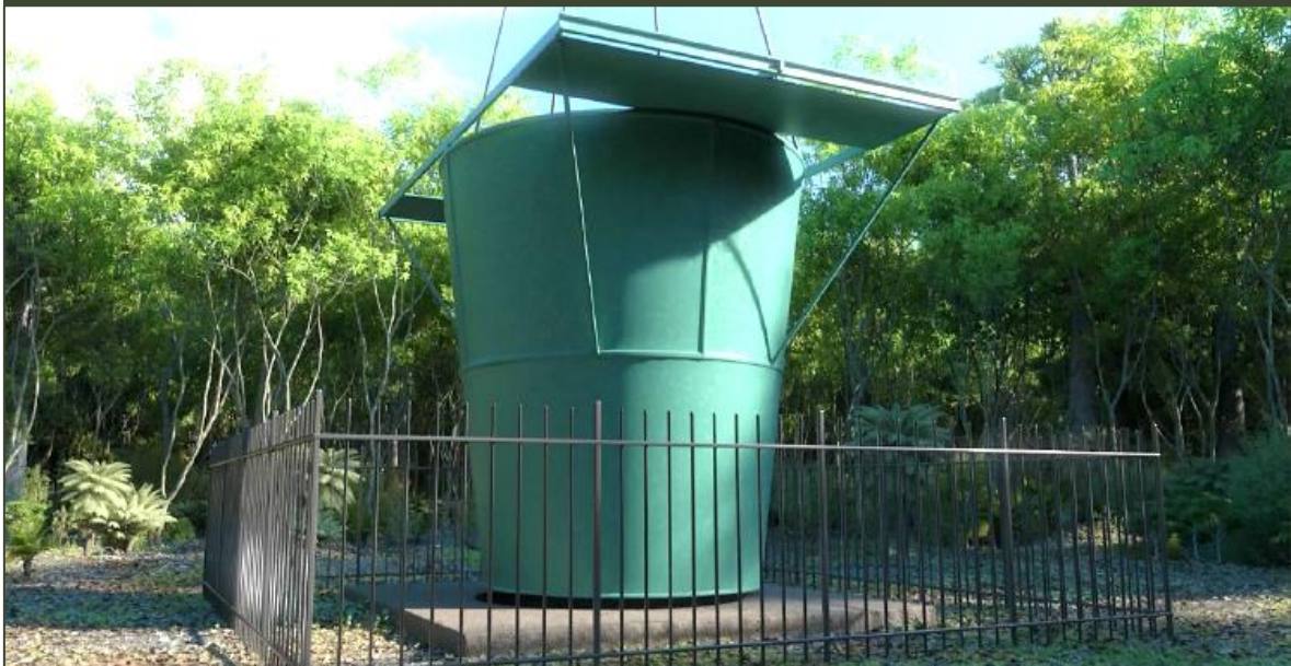
Figure 9: Design of surface infrastructure for ventilation raise (OGNZL supplied – note that exclusion fencing is not proposed)
