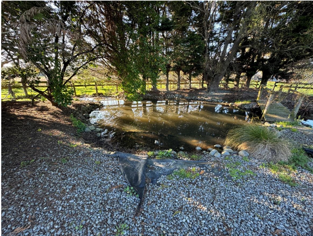
Figure 5: Ponded area with lining at end of wet water race reach.
