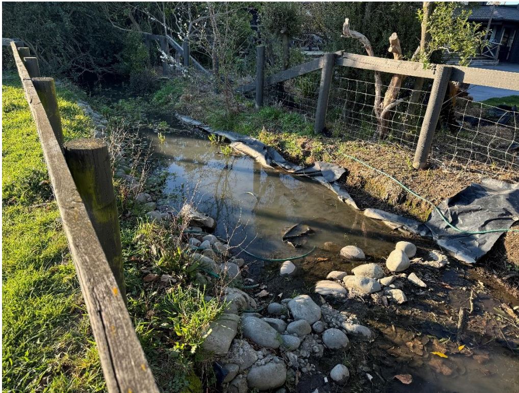
Figure 3: Wet reach along the 94 Barters Road driveway, with rock weir and lining.
