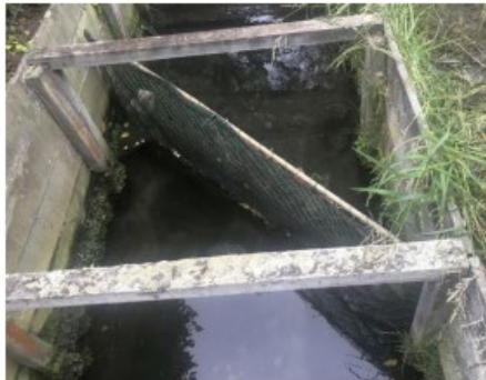
Example of a 'fence' type fish screen.
