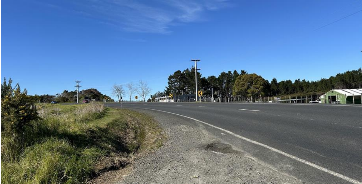
Figure 1: Sight line for Access 1 towards the east, showing grass within the legal road obstructing visibility
