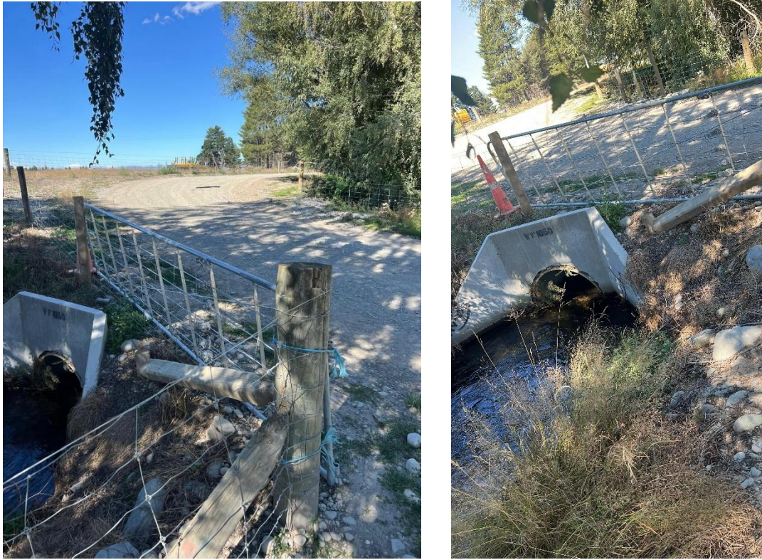
Figure 3.6: Road Crossing Water race over the culvert
