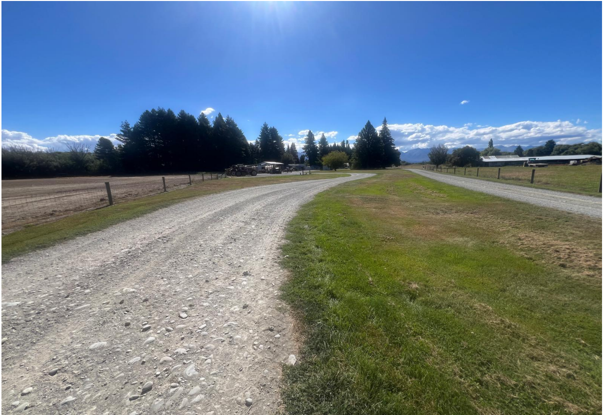
Figure 3.2: Local road unsealed typical view
