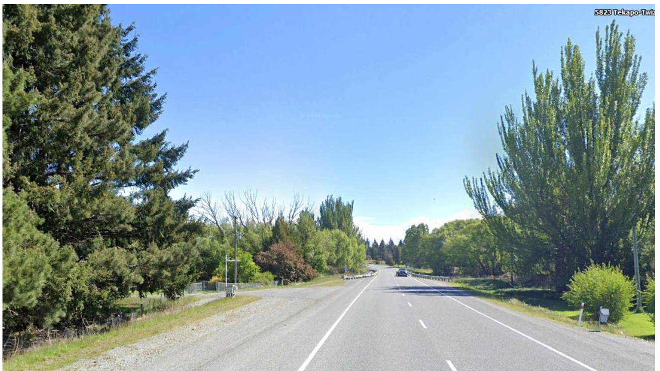
Figure 6.2: The site entrance looking towards Twizel – note sight lines and verge area
