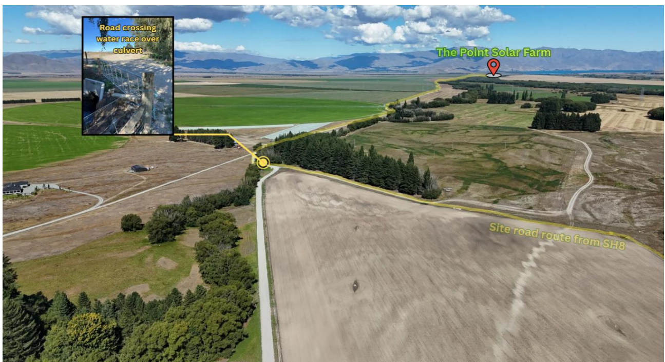
Figure 3.3: Local road unsealed typical view
