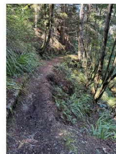
Track erosion and slippery pipe causing dangerous track conditions risking slip into gorge, with overtaking of exotic trees above
