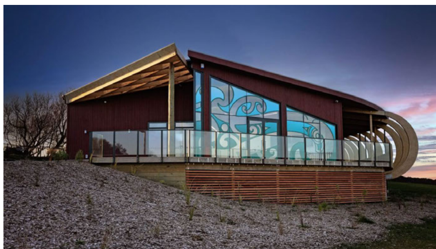
Figure 50 - The redeveloped Murihiku Marae in Invercargill, designed with the Waihōpai Rūnaka
