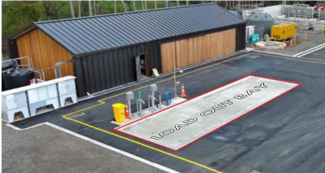
Figure 27 – An example of a bulk chemical load out bay
