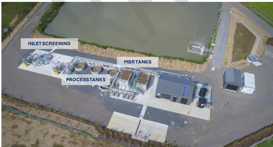
Figure 4: MBR treatment plant designed and built by Apex for Watercare
