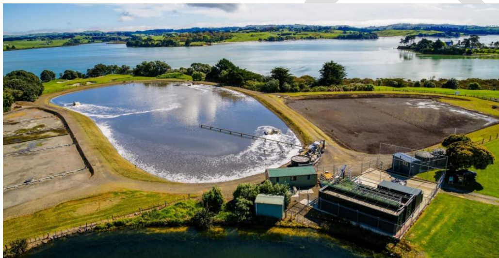
Figure 2410: Modular containerised MBR plant designed and built for Watercare
