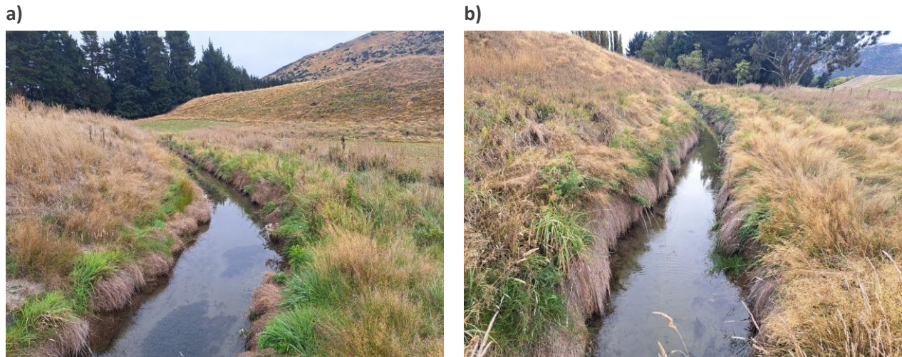
Figure 3. Examples of the water race within the site.
