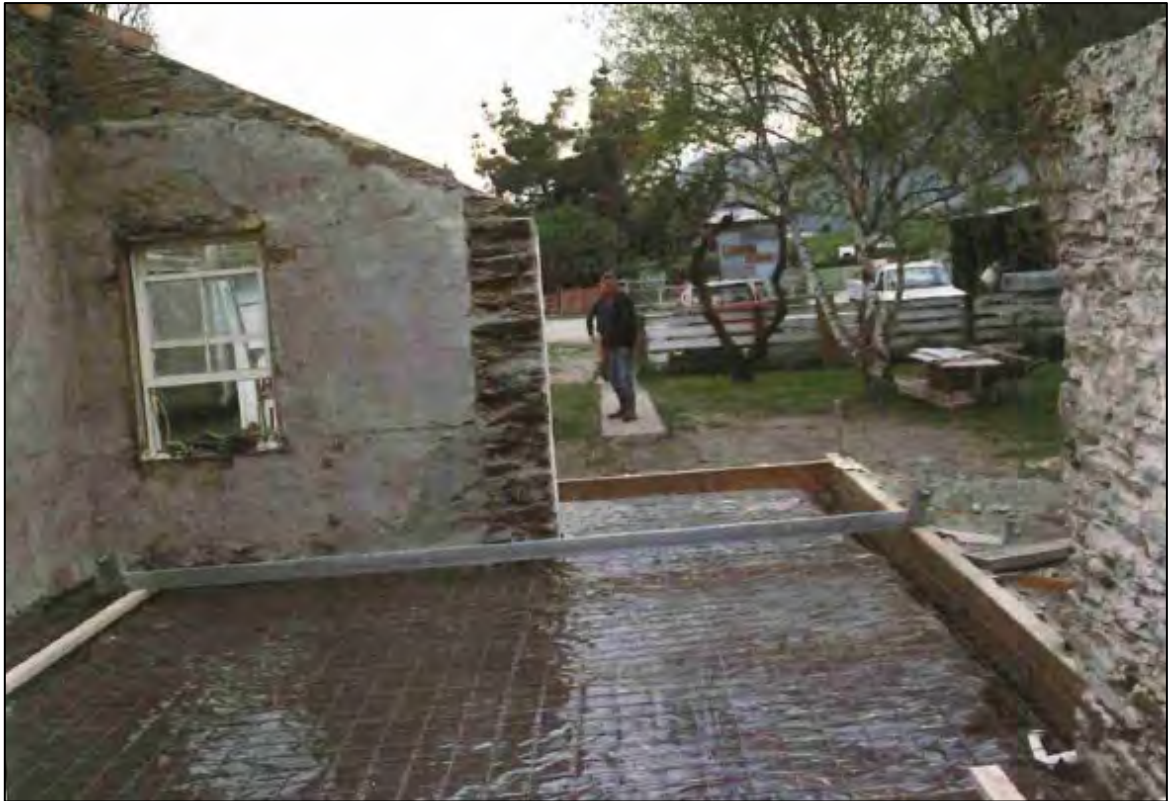
Figure 12. Rebuilding of kitchen, the walls and window are retained within the modern structure (Hamilton, 2016 p. 126).
