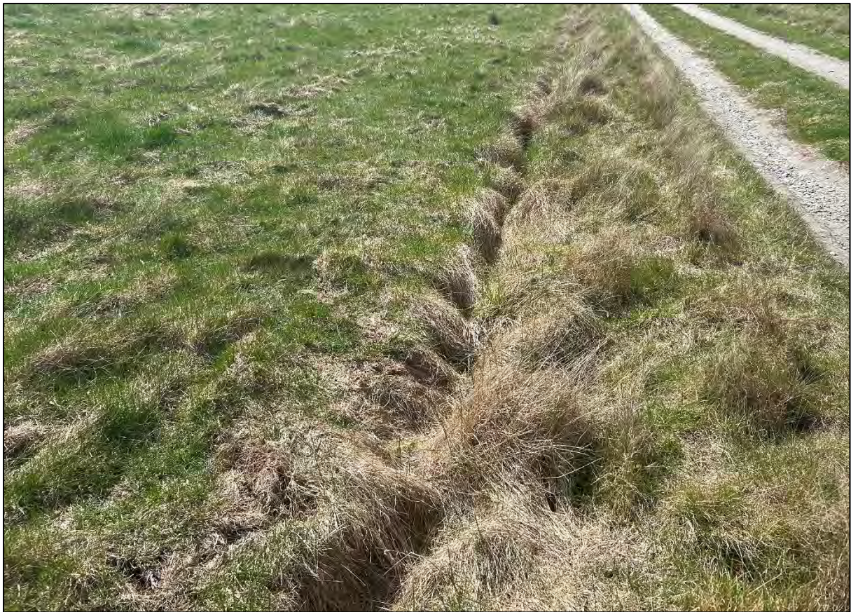
Figure 60. Potential ditch formation, to the east of main arrow irrigation race, facing north.
