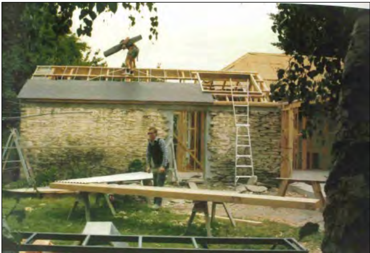
Figure 13. 20th century renovations revealing original roof shingles beneath current modern roof (Hamilton, 2016 p. 125).
