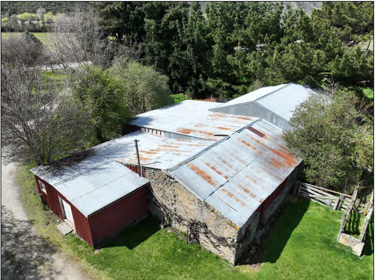
Figure 38. 19th century stables, with modern timber and steel extensions.
