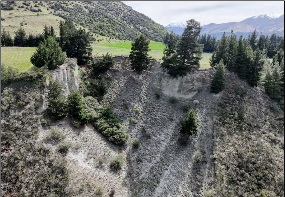
Figure 51. Eroded potential sluiced face facing toward flat plateau designated for development – (See Figure 28) – Section 25 Block IX.
