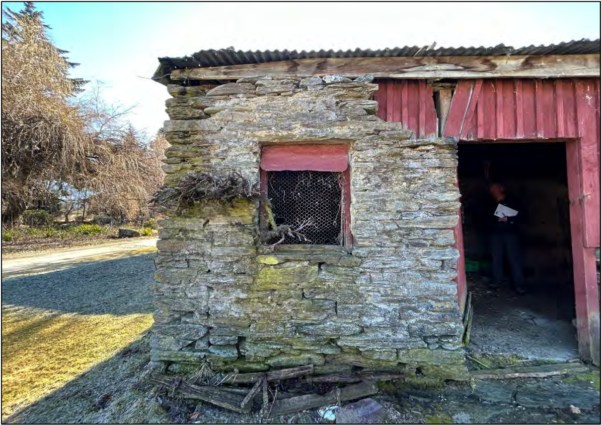
Figure 43. Facing north showing original stone wall.
