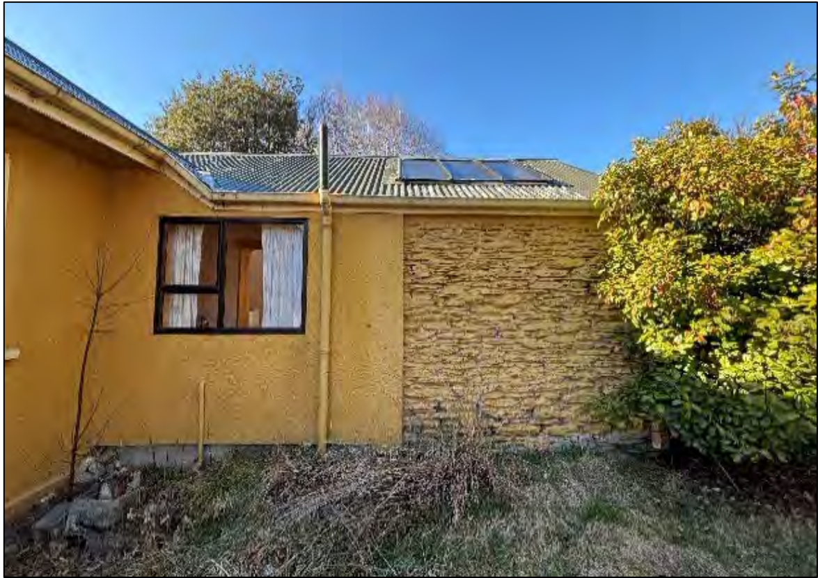
Figure 35 . Rear northwest elevation of David Jolly's stone shed.
